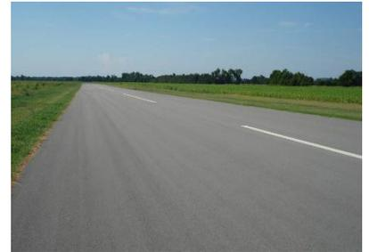
**RESULTS** The objective of this study was to assist in the construction of the UAV runway to develop a pavement that can be used as a test facility for evaluating environmental impact on pavement materials including but not limited to plant-mixed warm and hot mix asphalt pavements, high reclaimed asphalt pavement (RAP) and reclaimed asphalt shingles (RAS) mixes, asphalt surface treatments, pavement preservation treatments, 100% RAP cold mixes and aggregate bases with surface treatments.
