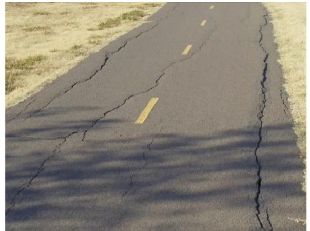
**Figure 1 Longitudinal Dry Shrinkage Cracks**
