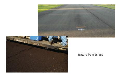
FIGURE 63 Example of large aggregates leaving tears in mat from being dragged by screed [*Source*: (*top*) Warren (2012); (*bottom*) Stroup-Gardiner (2014)].
