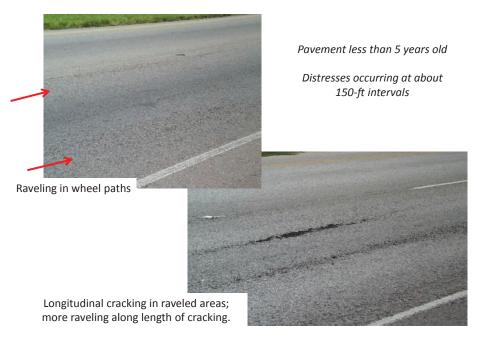
FIGURE 64 Example of how pavement distresses in segregated areas of the pavement progress with exposure to traffic and environmental conditions [*Source*: Stroup-Gardiner (2014)].
