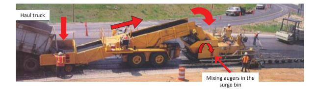
FIGURE 56 Example of a remixer in the surge bin in paver hopper [Source: Stroup-Gardiner (2014)].
