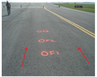
FIGURE 7 Example of longitudinal segregation, both sides [*Source*: Murphy (2012a)].
