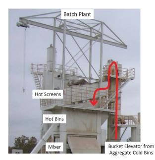
FIGURE 37 Components of a batch plant [*Source*: Stroup-Gardiner (2014)].
