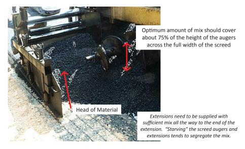
FIGURE 62 Example of depth of mix at auger [Source: Stroup-Gardiner (2014)].
