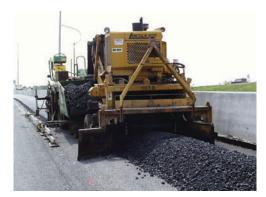
Pick-up devices may have only paddles to move the mix onto the internal conveyor or have a combination of augers and paddles.
