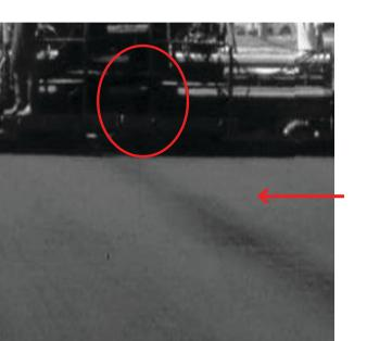
FIGURE 8 Example of centerline longitudinal segregation under gear box [*Source*: Stroup-Gardiner (2014)].
