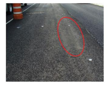
FIGURE 5 Example of random segregation (separation of binder and stone) in SMA [*Source*: Stroup-Gardiner (2014)].
