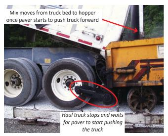
FIGURE 47 Transferring asphalt mix to the paver hopper [*Source*: Stroup-Gardiner (2014)].
