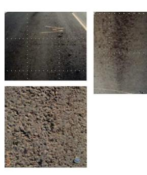
FIGURE 10 Example of moderate level of segregation [*Source*: Gavin and Heath (2002)].
