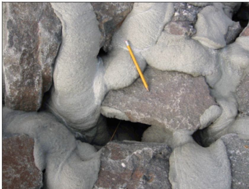
Figure 14.7-A — CLOSE-UP VIEW OF PARTIALLY GROUTED RIPRAP
