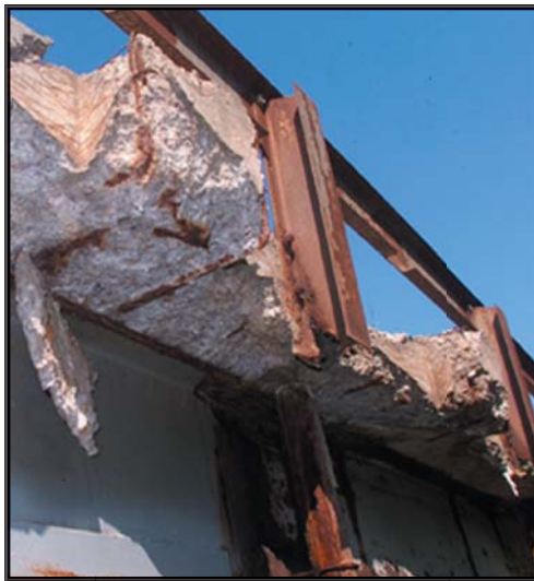
Crumbling barrier walls
