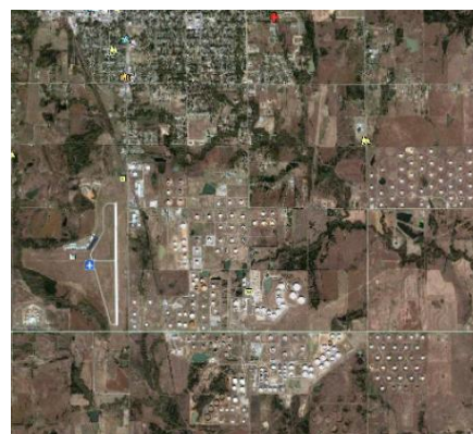
FIGURE 26: AERIAL VIEW-CUSHING TANK FARM
