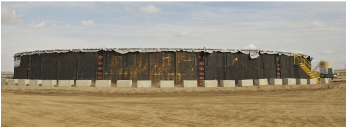
Figure 1 Outside of a double-walled above-ground storage tank holding produced water in North Dakota (Williams County)
