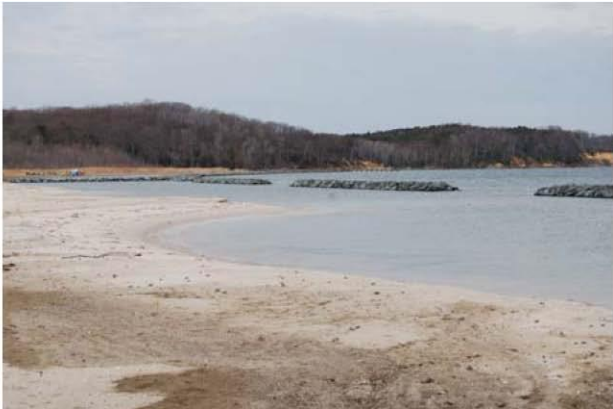
Newly-nourished beach with segmented breakwaters in Chesapeake Bay in right of photos.
