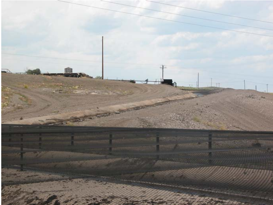
VIEW OF "CEMENT PIT" PRIMARY PIT INPUT WITH NETTING TO PROTECT WILDLIFE
