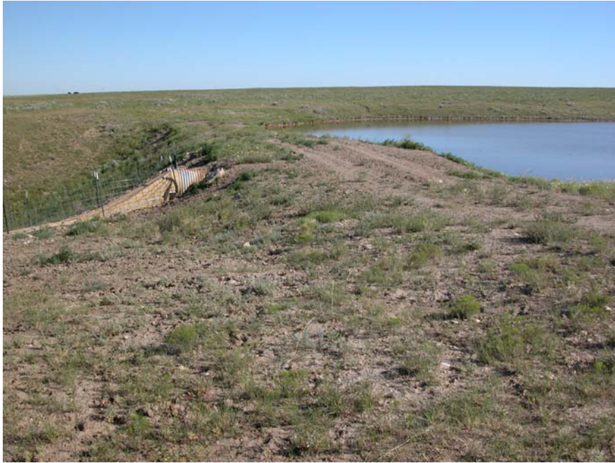
VIEW OF STOCK POND DAM WITH PRIMARY SPILLWAY PIPES
