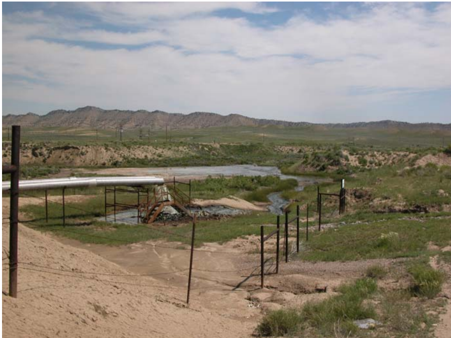
VIEW OF SECOND PIT'S DISCHARGE TO BUFFALO CREEK
