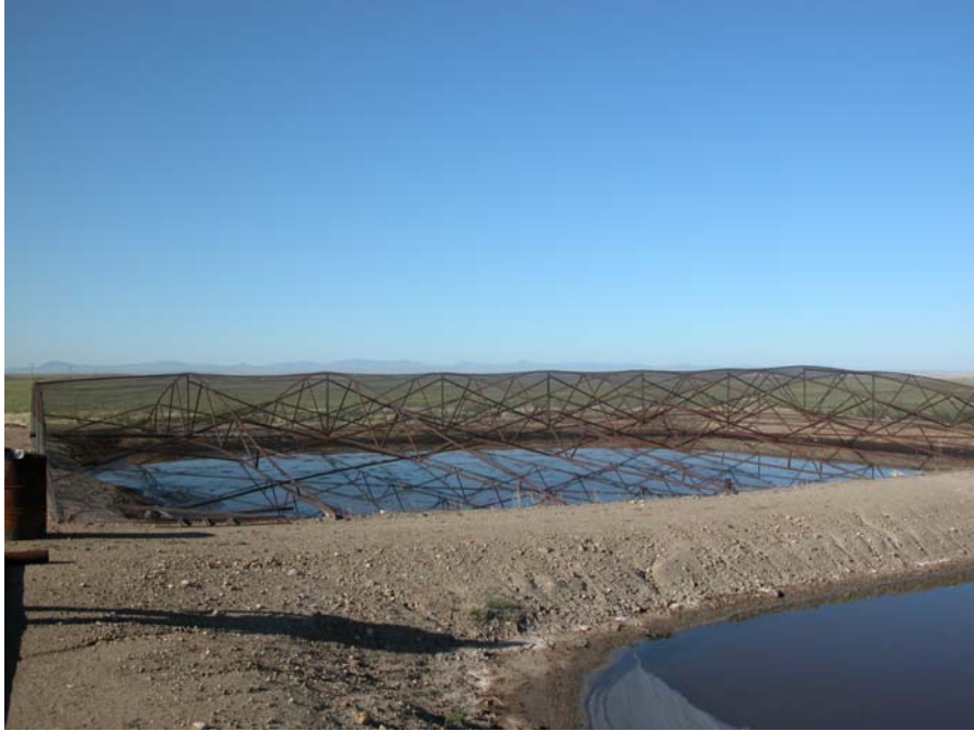
VIEW OF SECONDARY SEPARATION PIT ENCLOSED WITH A FENCE AND A CATTLE GUARD
