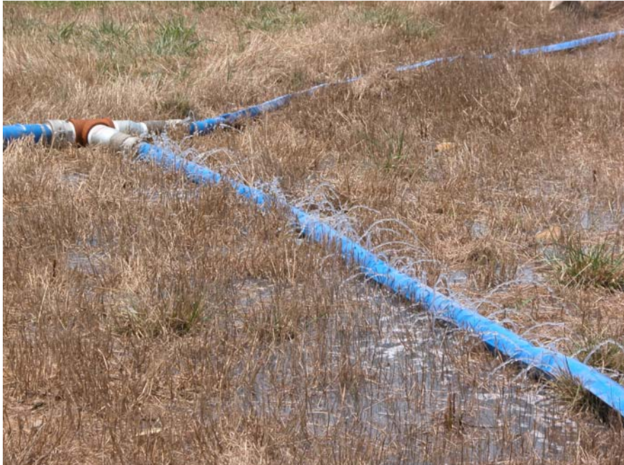
VIEW OF A FLOOD IRRIGATION SYSTEM AS WATER IS DRAINED FROM THE STORAGE TANK
