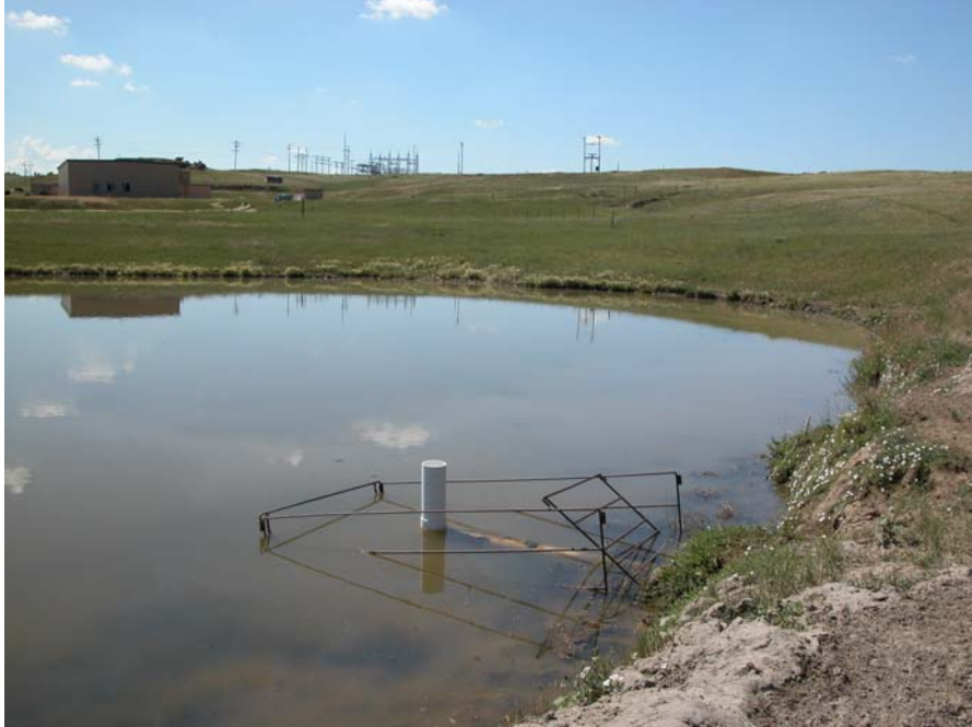
VIEW OF SECONDARY PIT T-SIPHON TO PREVENT OIL FROM DISCHARGING
