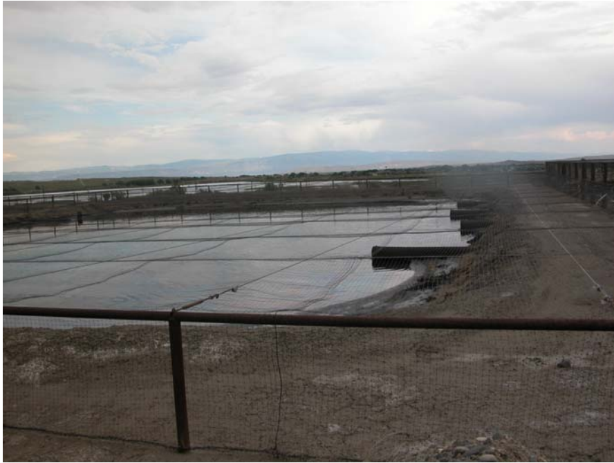
VIEW OF SECONDARY PIT WITH NETTING WHERE THE WATER IS POLISHED FURTHER WITH T-SIPHONS
