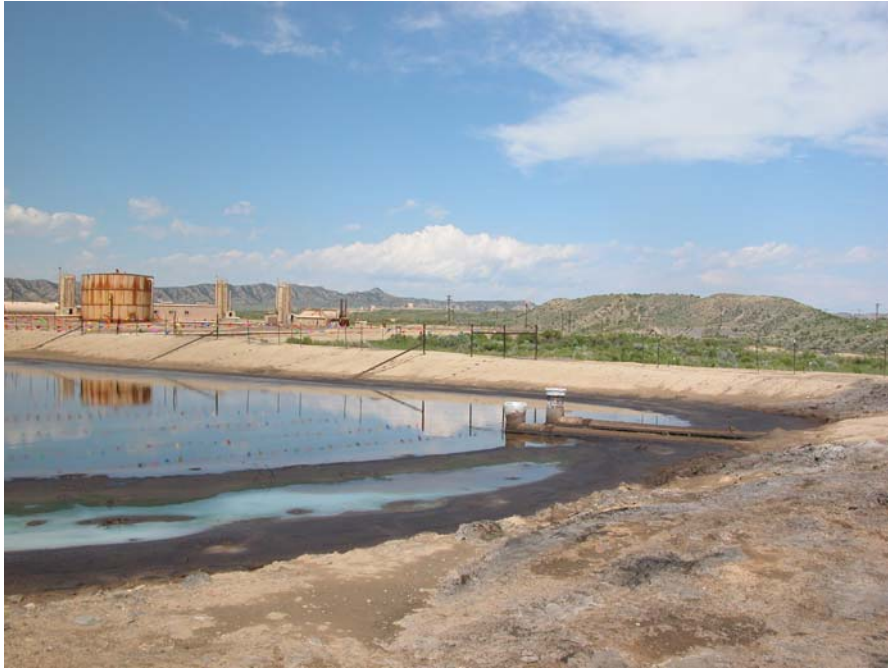
VIEW OF SECOND PIT WITH TWO T-SIPHONS TO PREVENT OIL FROM DISCHARGING
