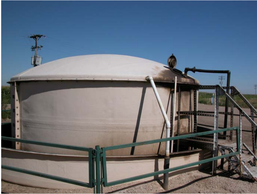
VIEW OF A TYPICAL STORAGE TANK AT A WELL HEAD
