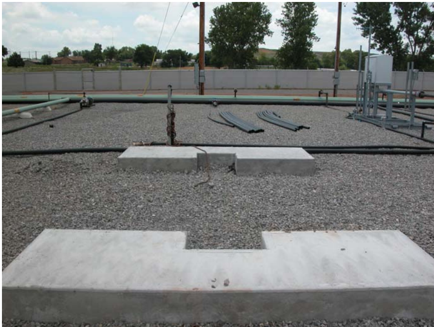
VIEW OF A FOUNDATION THAT HAS BEEN CONSTRUCTED FOR AN ADDITIONAL 3 PHASE SEPARATOR
