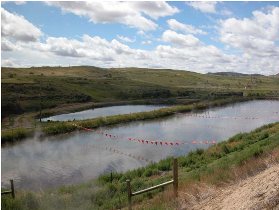
VIEW OF SECONDARY AND TERTIARY PITS PRIOR TO DISCHARGE TO TEAPOT CREEK
