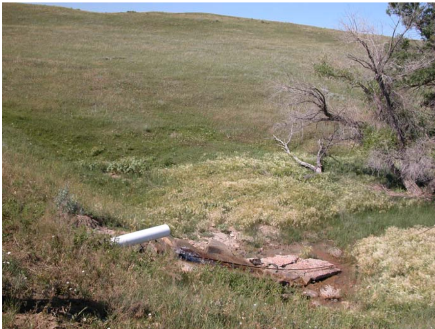
VIEW OF SECONDARY PIT DISCHARGE TO BELL CREEK
