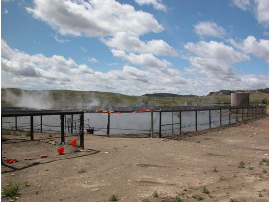
VIEW OF STEAM GENERATED FROM A NETTED PRIMARY SEPARATOR PIT
