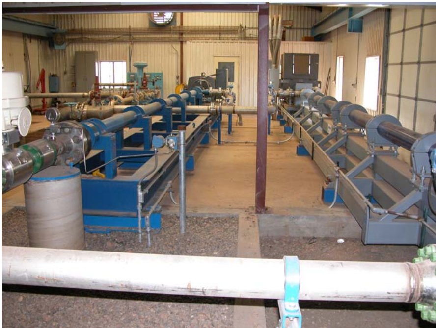
VIEW OF PUMPING UNITS THAT PUMP WATER TO INJECTION WELLS
