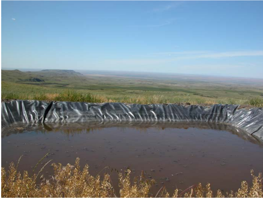
VIEW OF A LINED PIT ADJACENT TO A WELL HEAD
