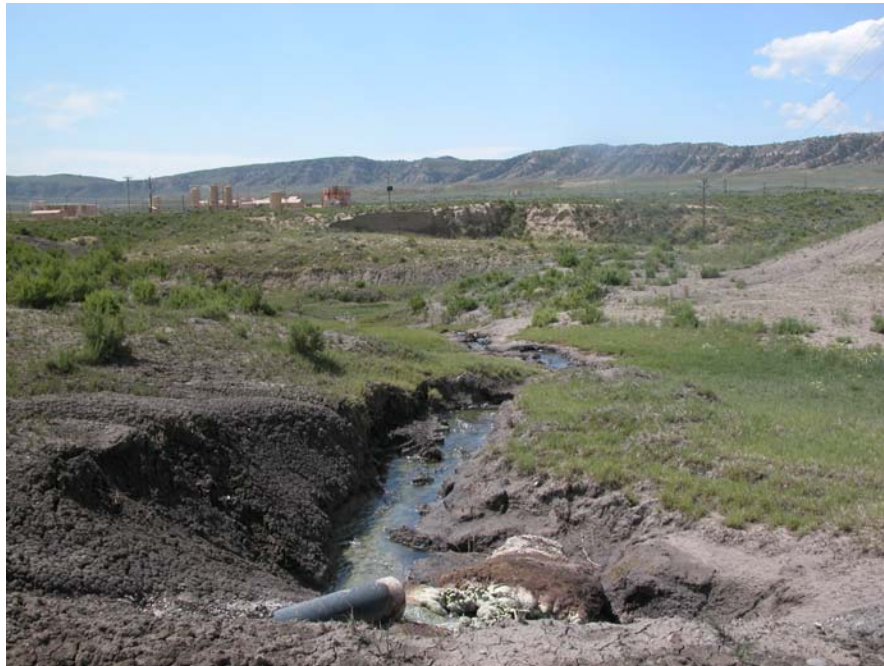
VIEW OF FIRST PIT'S DISCHARGE TO BUFFALO CREEK
