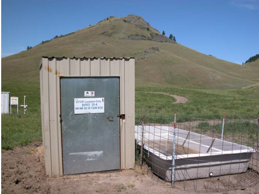
VIEW OF A WELL HEAD WITH A TANK ADJACENT TO IT TO HOLD PRODUCED WATER
