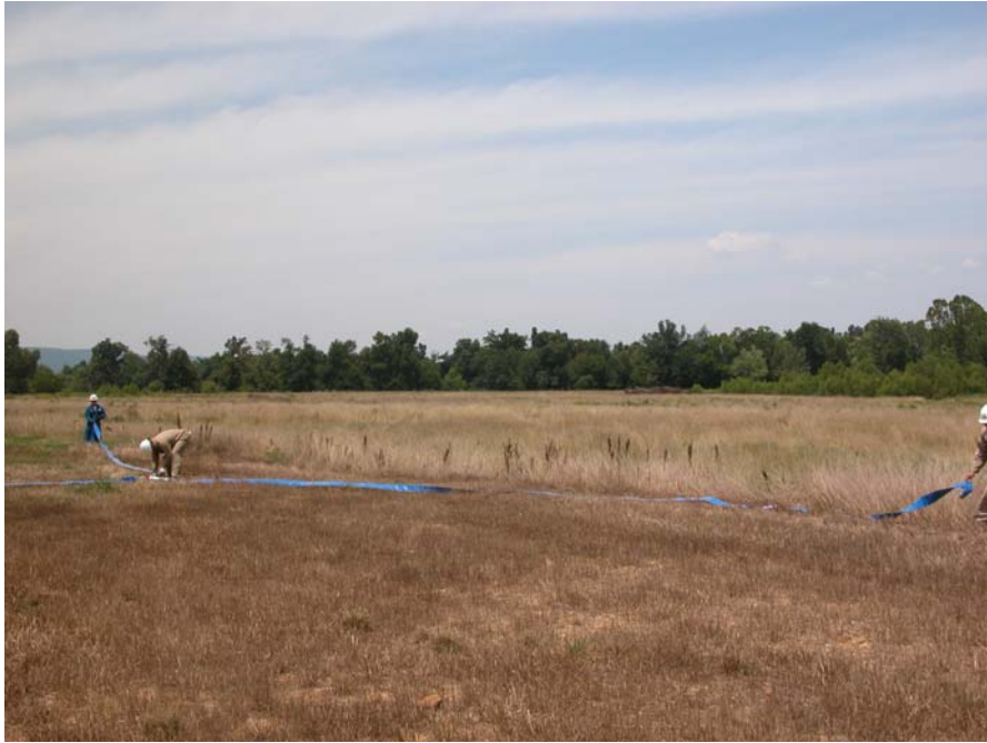
VIEW OF THE DEPLOYMENT OF TEMPORARY FLOOD IRRIGATION SYSTEM
