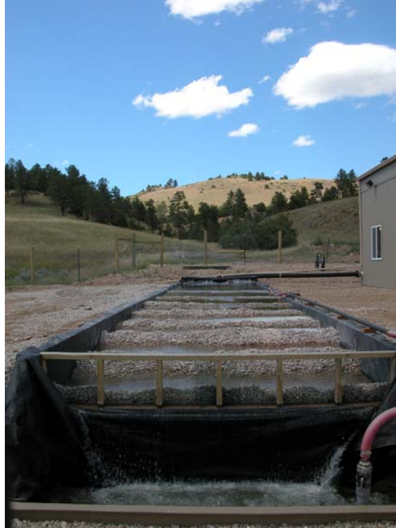
CLOSER VIEW OF THE AERATOR PRIOR TO DISCHARGE TO RETENTION PIT
