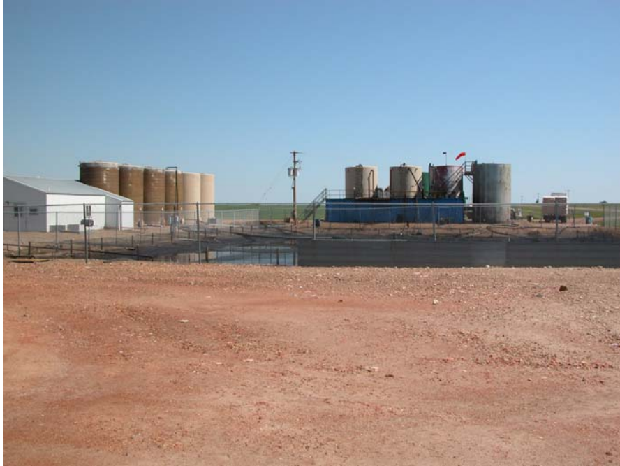
VIEW OF INJECTION WELLHEAD AT NANCE
