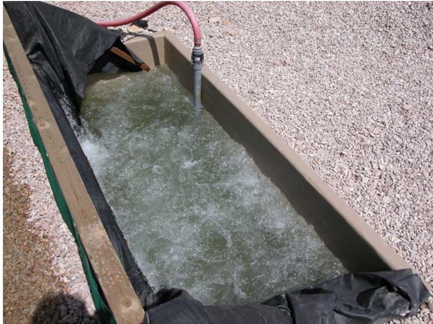
CLOSER VIEW OF THE AERATOR PRIOR TO DISCHARGE TO RETENTION PIT
