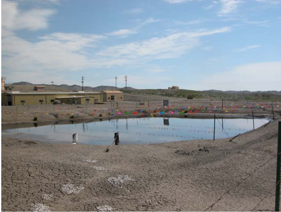
VIEW OF FIRST PIT WITH T-SIPHON TO PREVENT OIL FROM DISCHARGING
