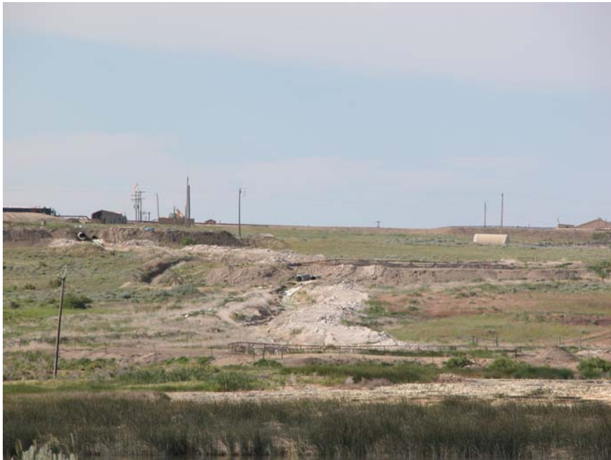
CLOSER VIEW OF PIT SYSTEM THAT DISCHARGES TO CUSTER LAKE
