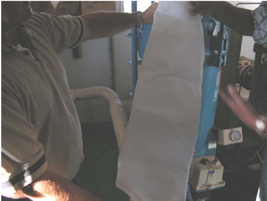
VIEW OF THE SOCK FILTER THAT REMOVES SOLIDS FROM THE WATER BEFORE REINJECTION
