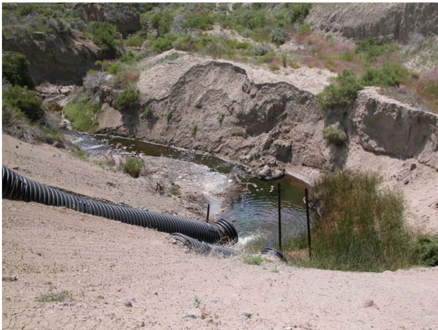
VIEW OF SECONDARY PIT DISCHARGE TO SILVER TIP CREEK
