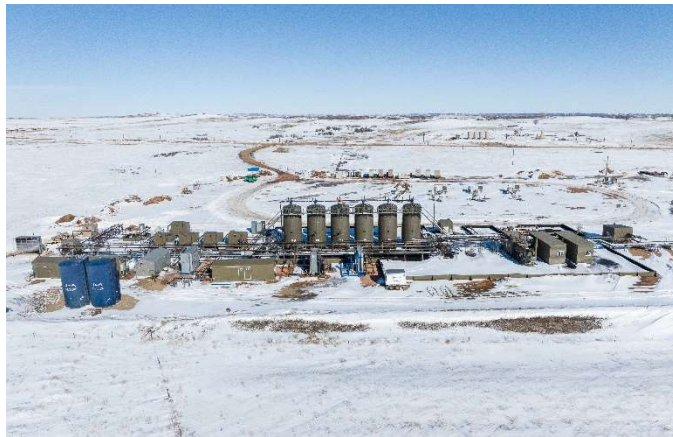
Figure 2: LEAF Production Facility in the Field.
