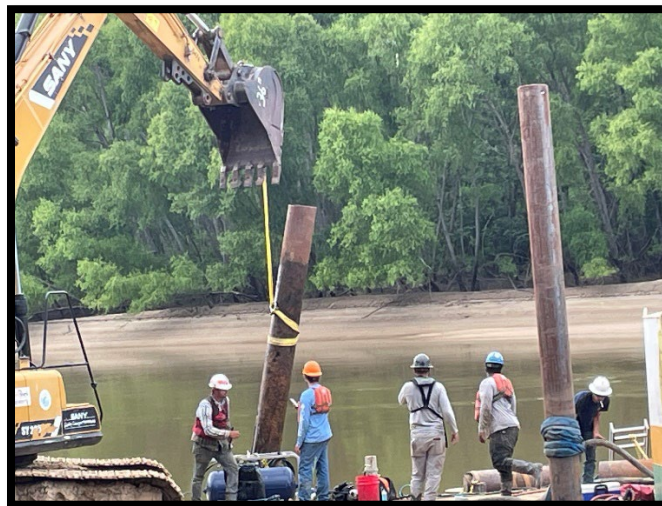
Figure 5: Neches River in Big Thicket National Preserve—removing surface casing
