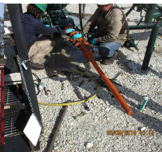
Valve Recovery Plug Installation
