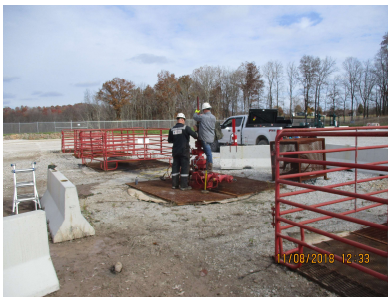
Back Pressure Valve Installation
