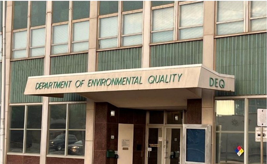
Figure 2. The street façade of DEQ’s central offices, located at 707 N. Robinson Ave, OKC.
