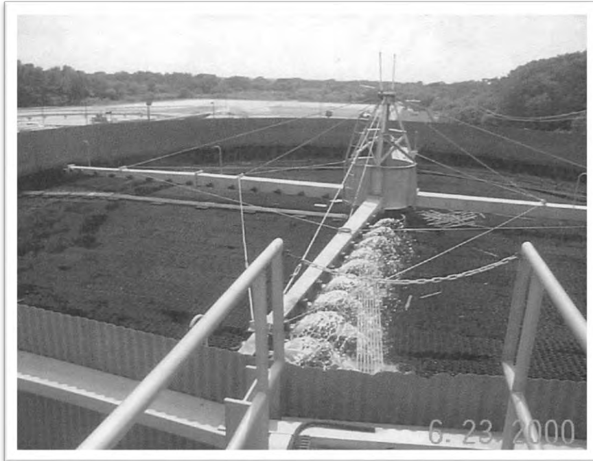
Trickling filter with plastic media.
