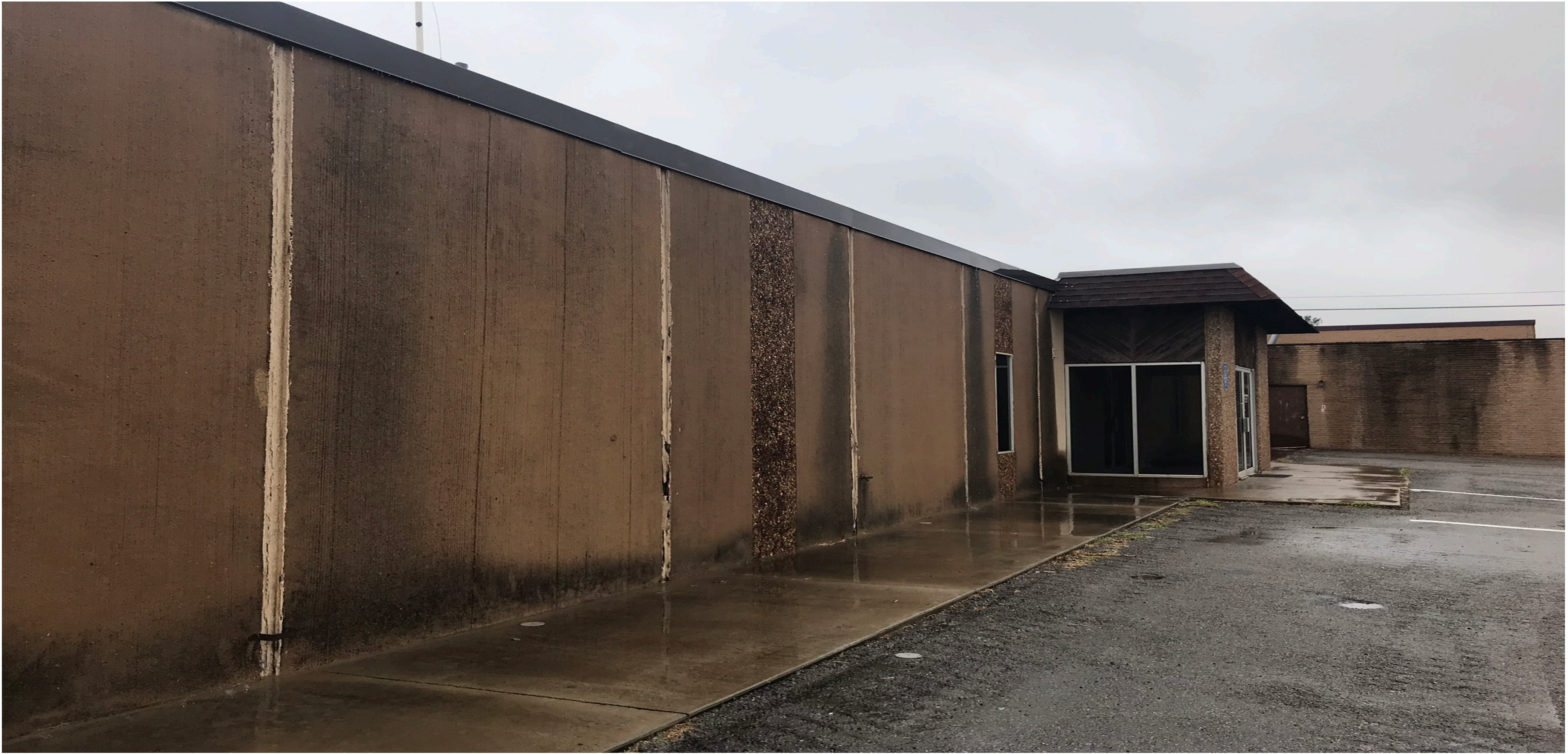
Police Building - ACM Wall Expansion Joint Texture/Barrier - round the building
