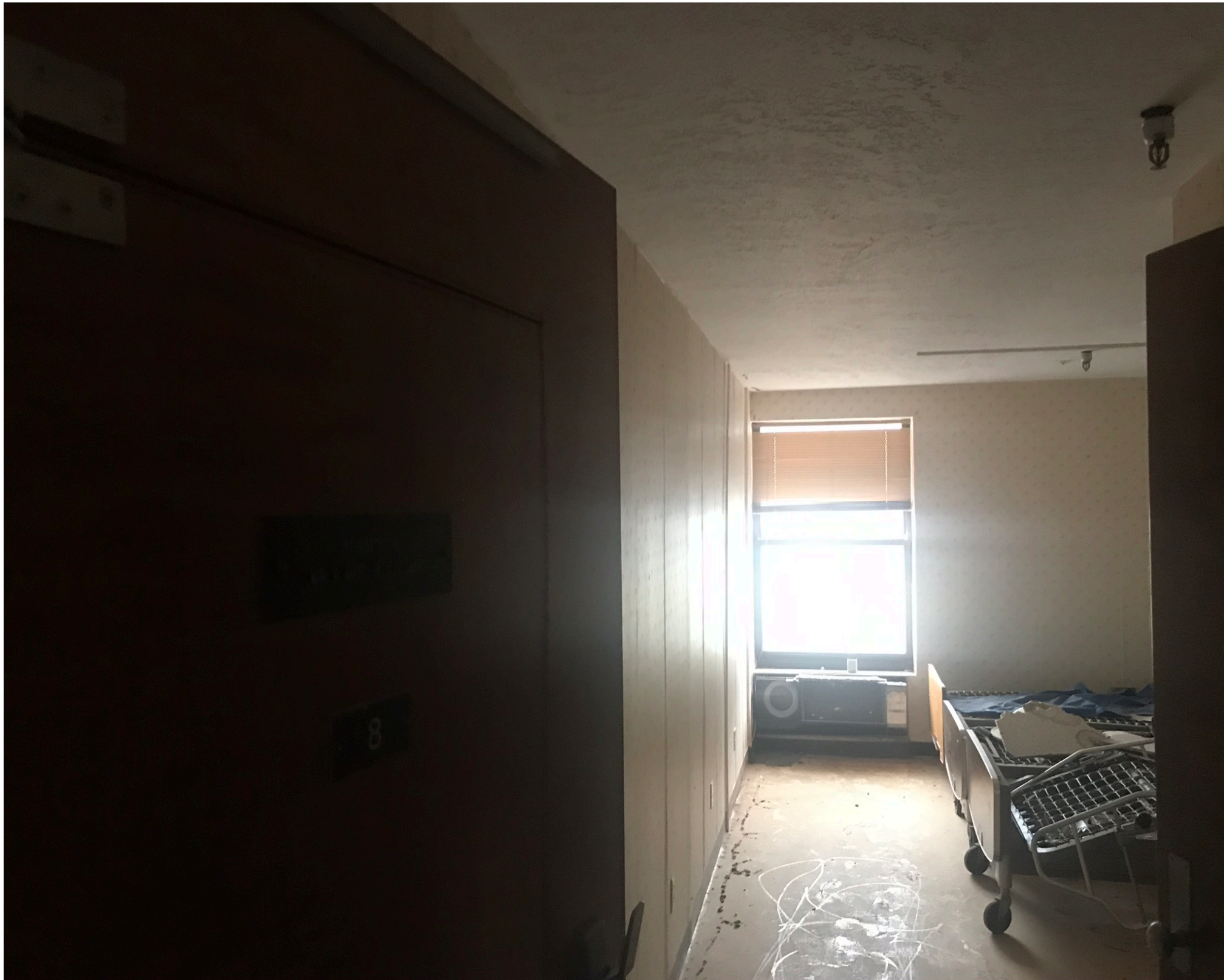
Bldg. 7 Room 6&8 - ACM - Walls/ceiling/sheet flooring
