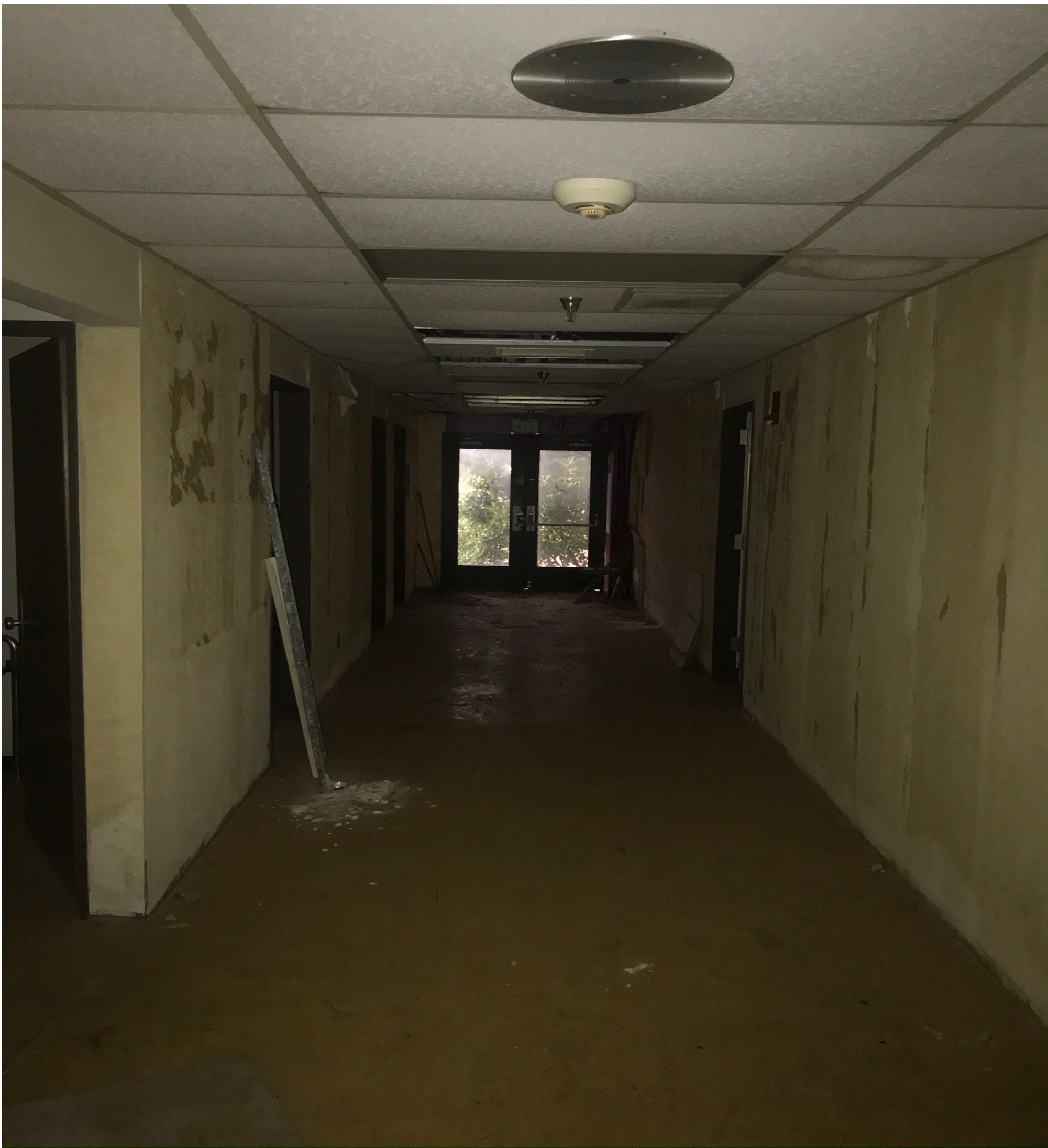
Bldg. 7 Room 20 Hallway - west: ACM - Sheet flooring & texture/joint compound wall systems
