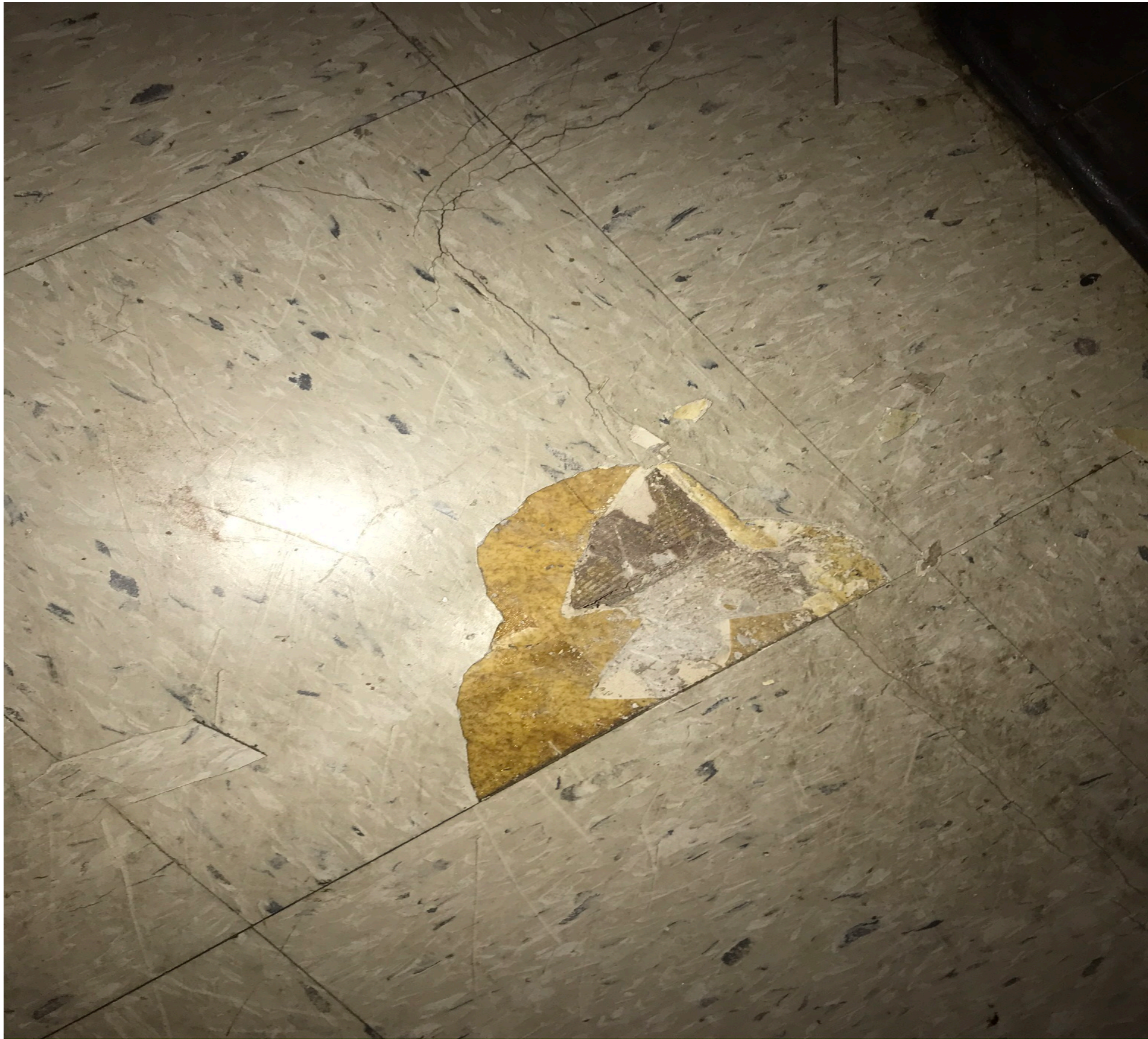
Room 1 & Room 123 Hallway - ACM sheet flooring beneath the floor tiles in all rooms/hallway throughout the nursing home (Building 1-3)
