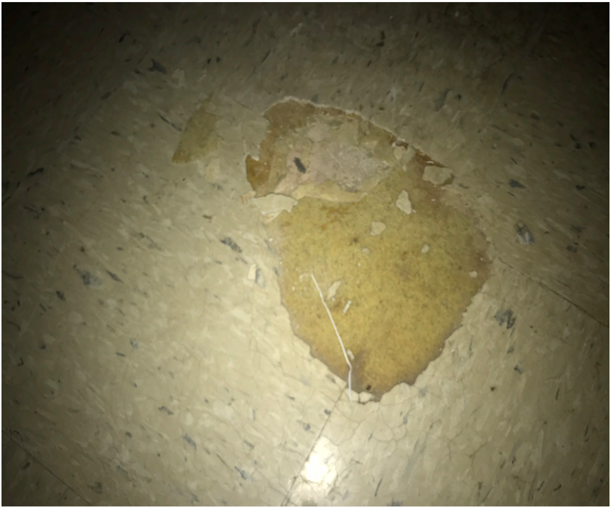
Room 1 & Room 123 Hallway - ACM sheet flooring beneath the floor tiles in all rooms/hallway throughout the nursing home (Building 1-3)
