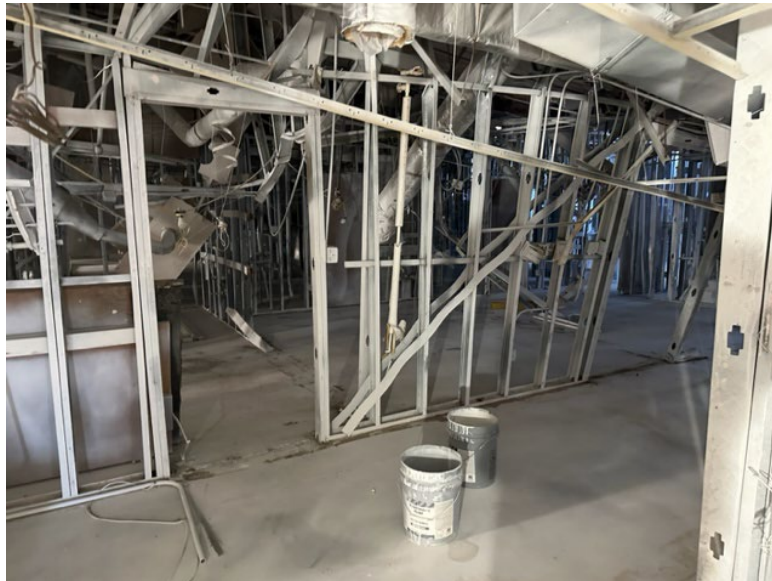
PHOTO # 2 – View of SW area after abatement and lockdown.
