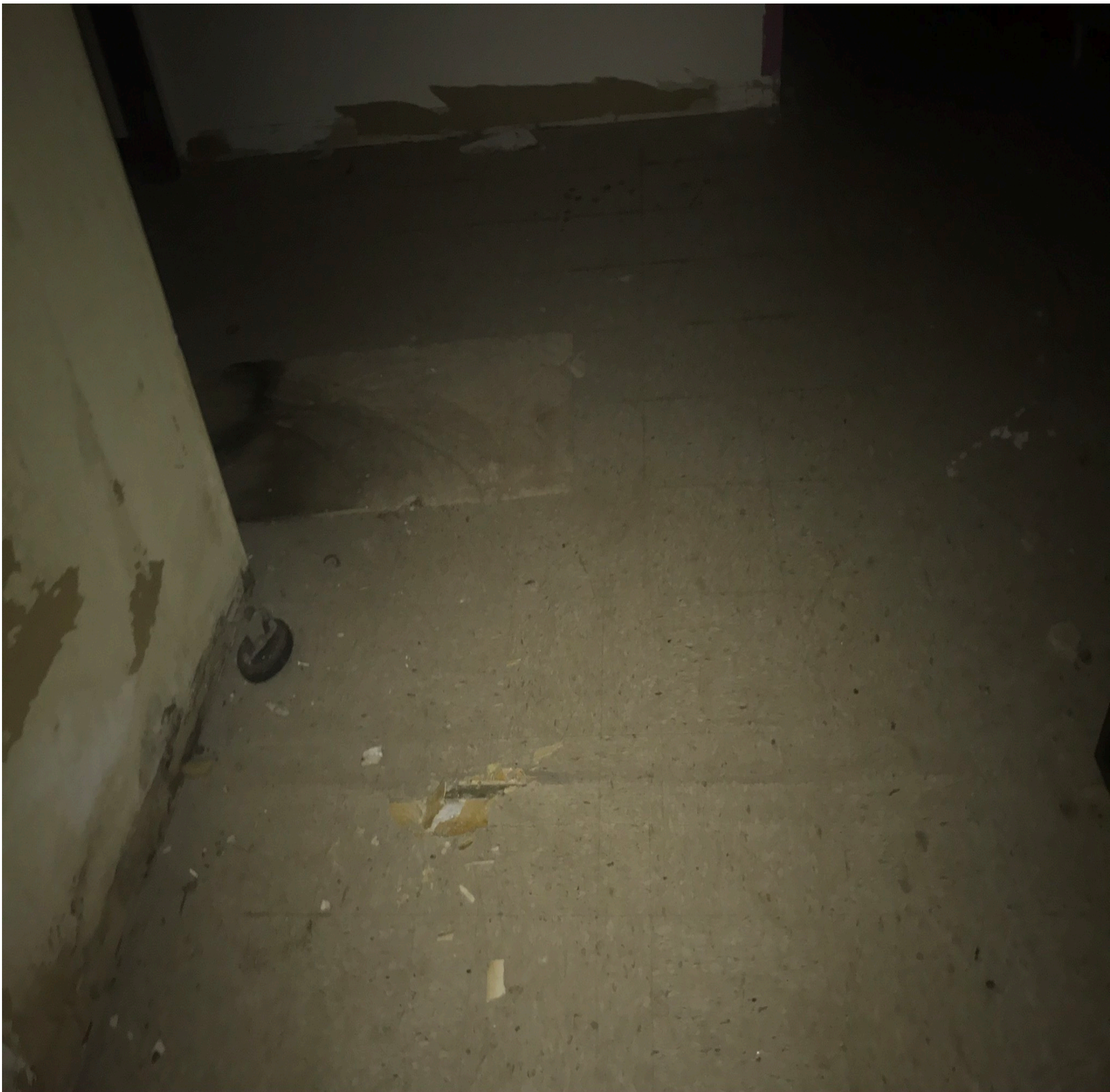
Bldg. 7 Room 34 Hallway - ACM: Sheet flooring beneath floor tiles throughout bldg. 7
