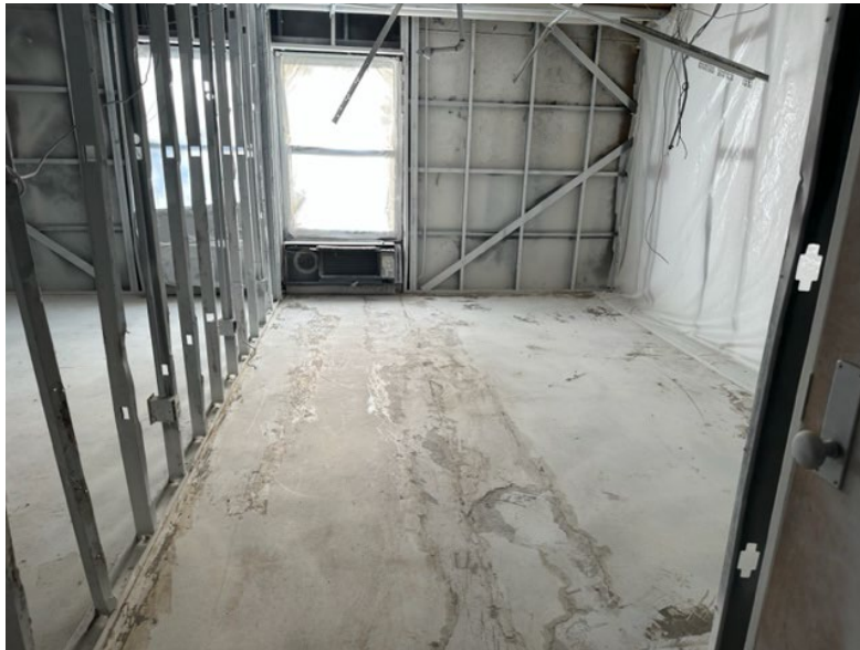
PHOTO # 4 – View of SE area after abatement and lockdown.
