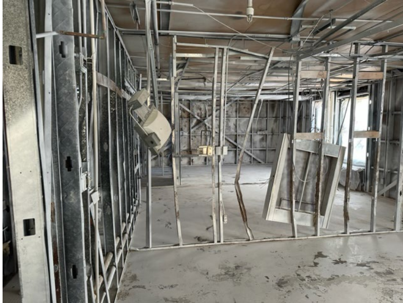
PHOTO # 1 – View of NW area after abatement and lockdown.
