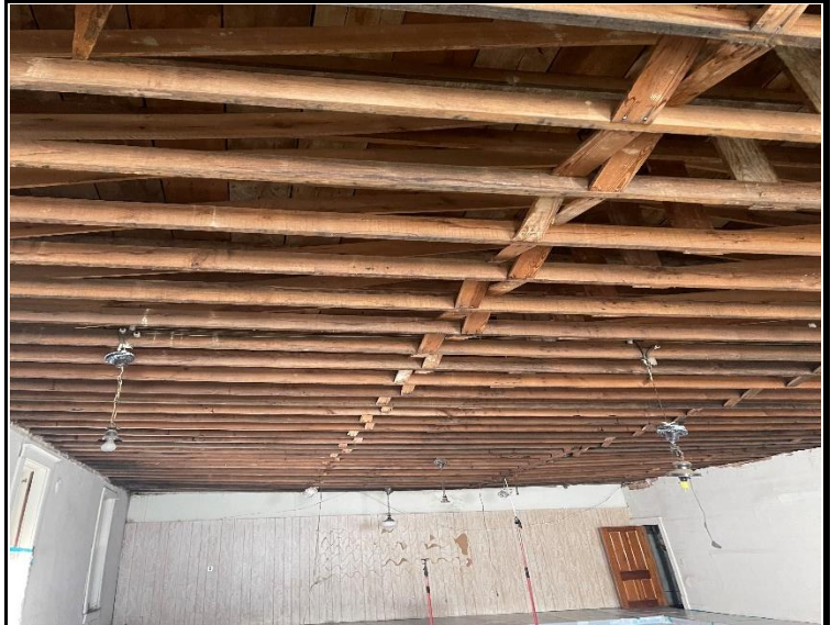
Photo 18: Thomas Apartments LBP Abatement Progress Room 1 Ceiling After Removal
