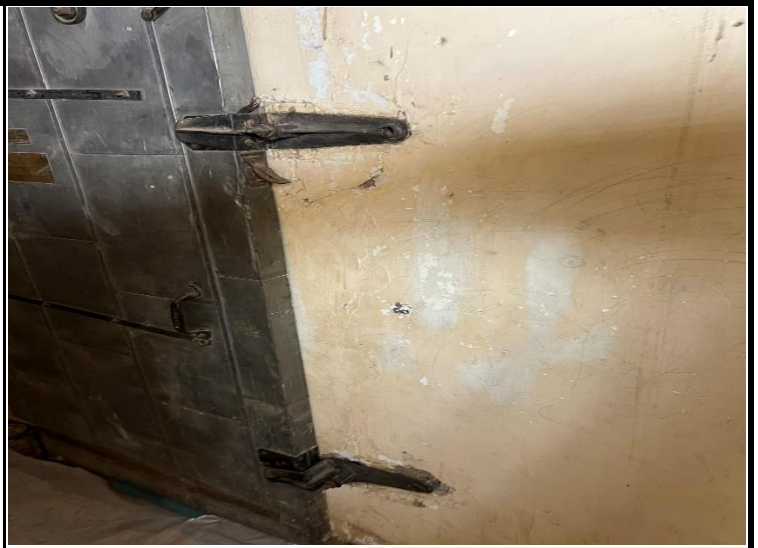
Photo 20: Thomas Apartments LBP Abatement Progress Fier Door After Door Component Scrape
