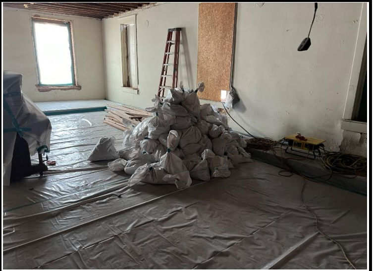
Photo 2: Thomas Apartments Abatement Progress, LBP Debris Room 1 North Wall Demo
