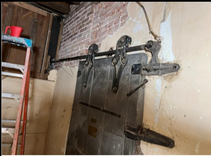
Photo 19: Thomas Apartments LBP Abatement Progress Fier Door After Door Component Scrape
