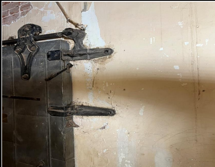
Photo 21: Thomas Apartments LBP Abatement Progress Fier Door After Door Component Scrape
