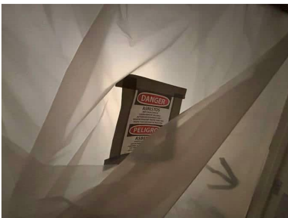
Photo 3 Southern front desk area during containment set up
