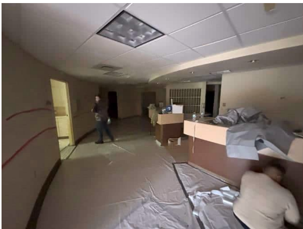
Photo 1 Hallway area during containment set up
