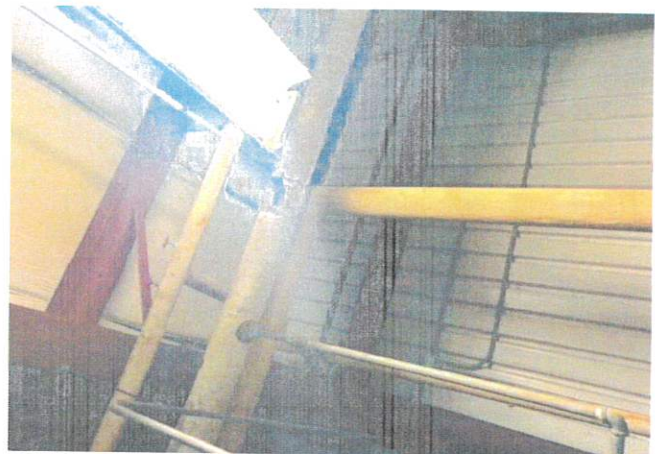
Asbestos containing insulation on piping
