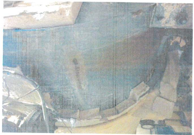
Boiler 1 exposed and missing Asbestos Insulation
