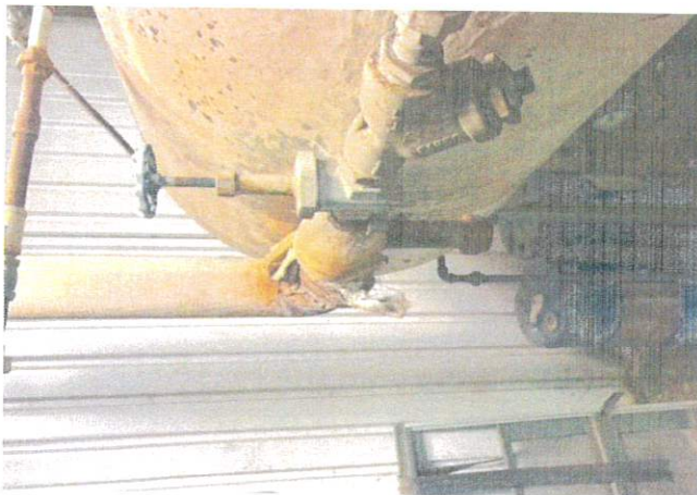
Deteriorated Asbestos containing material on pipe
