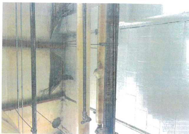
Possible roof leak above deteriorated asbestos material
