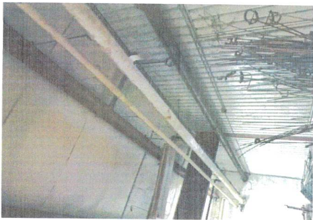
Overall of Asbestos containing material on piping
