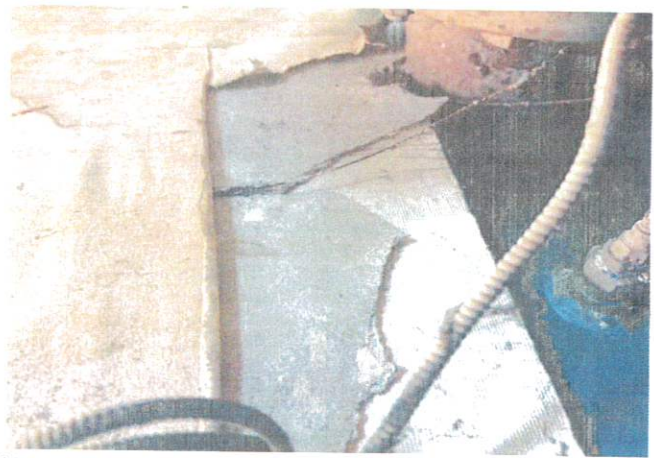
Close up of asbestos containing material on Boiler 1
