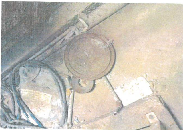
Loose Asbestos containing material on floor below Boiler
