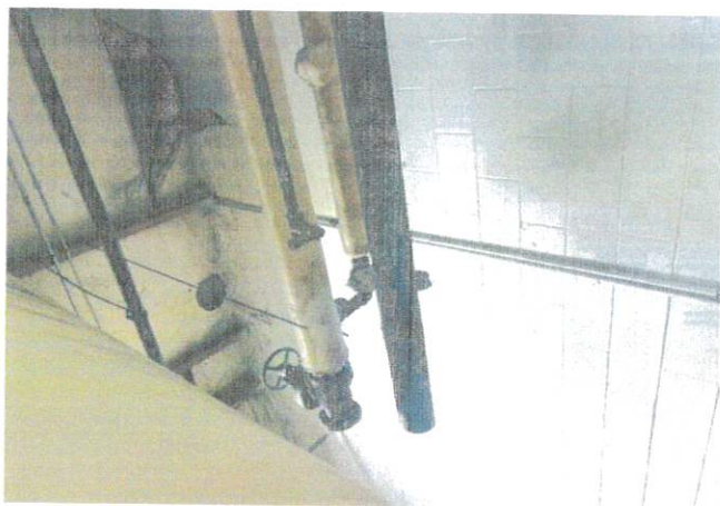
Deteriorated Asbestos containing material
