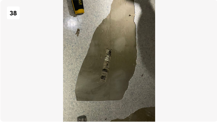
Black Mastic beneath the linoleum in the ER Hallway
