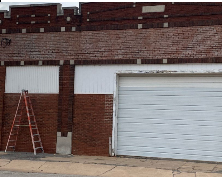
Photo 6: Exterior side D paint on brick
