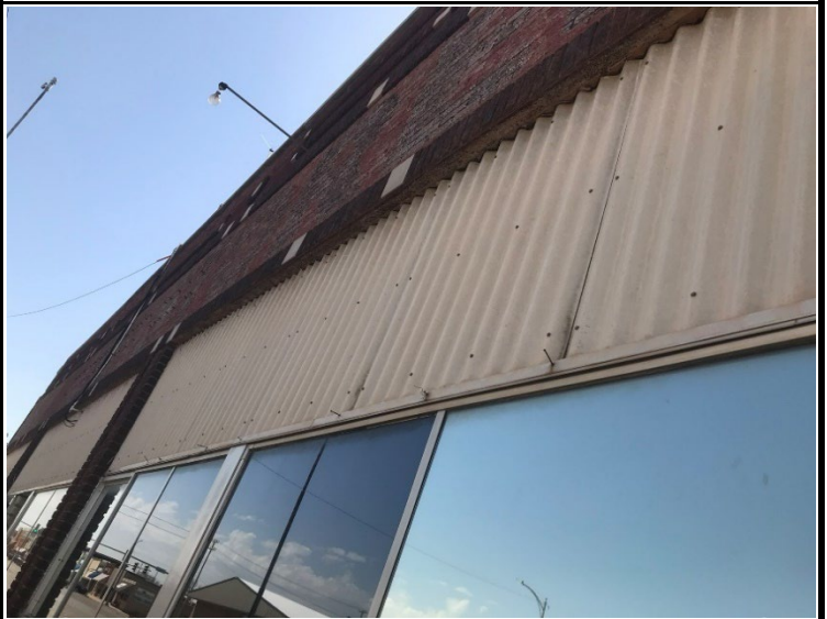
Photo 6: Exterior Wall Transite
