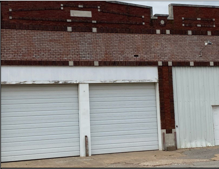
Photo 2: Exterior side D paint on brick
