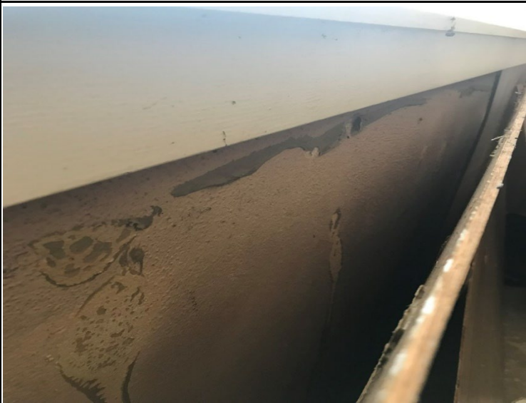
Photo 3: RM2- Gray Wall Mastic on East Wall
