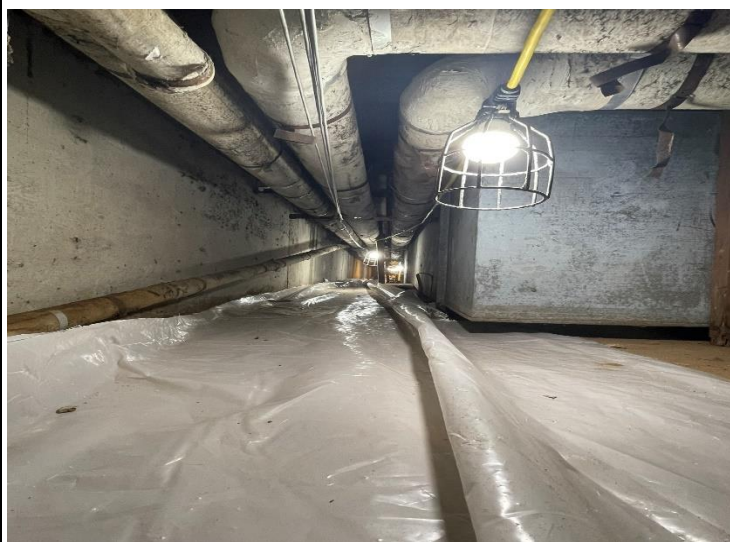
Photo 3: Parkside - in Tunnel - TSI Prep
