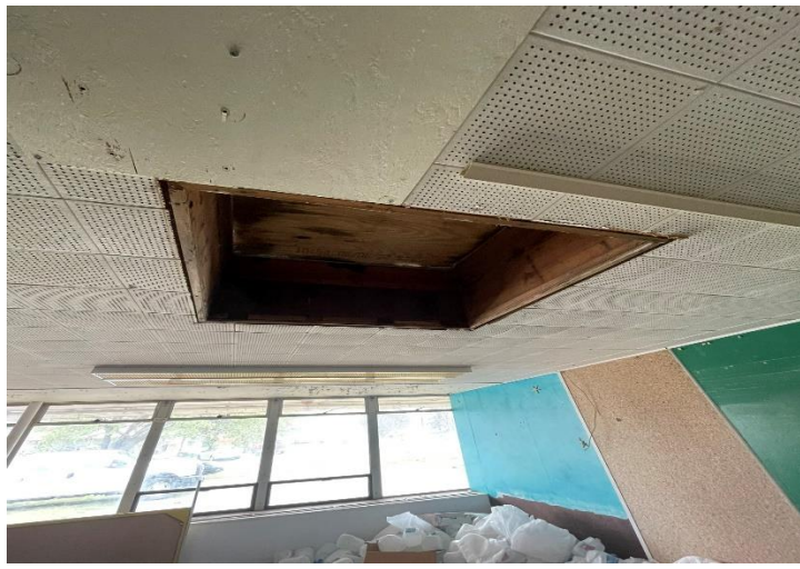
Photo 1: Parkside - South Building - Transit Pannel Abated
