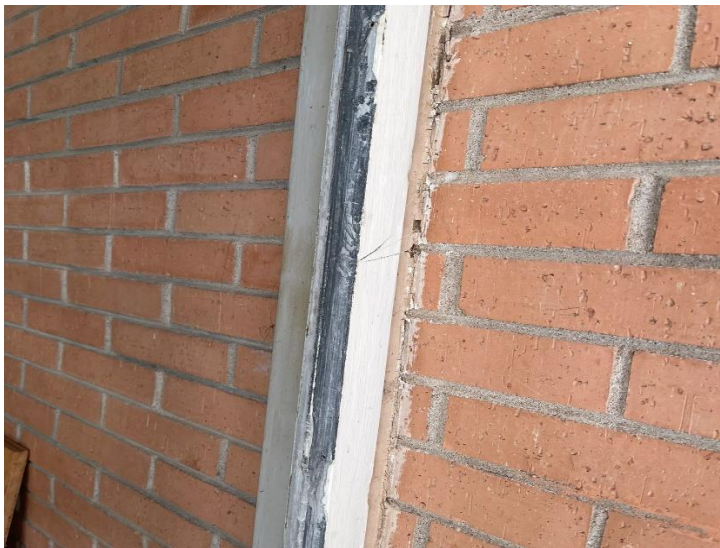
Photo 3: Parkside - North Building - Window Glaze Abated
