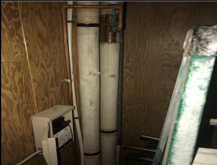
Photo 5: Asbestos Containing Pipe Insulation Building B Room 13
