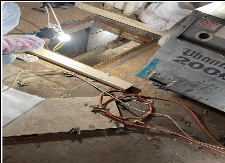
Photo 2: Parkside - Man Hole in South Building - TSI Prep
