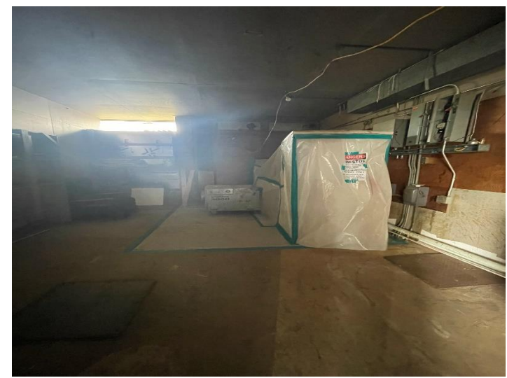
Photo 3: Parkside - South Building - Change Room - TSI
