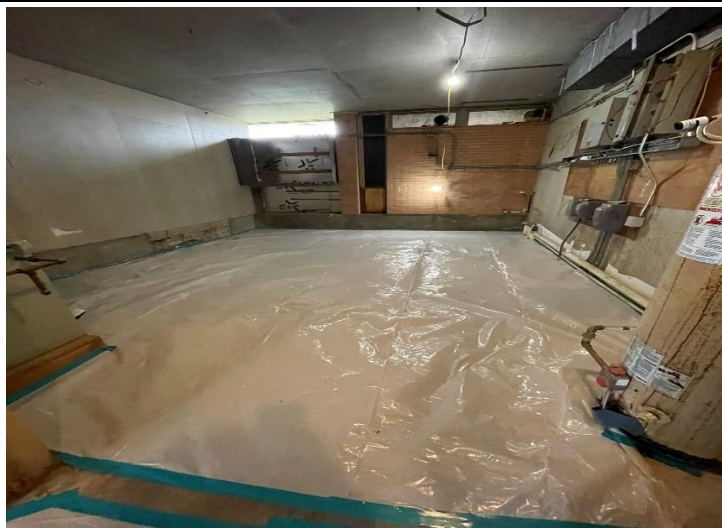
Photo 1: Parkside - South Building - Transit Prep
