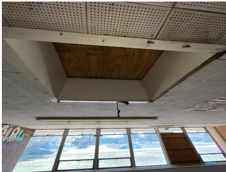
Photo 5: Parkside - South Building - Transit Pannel
