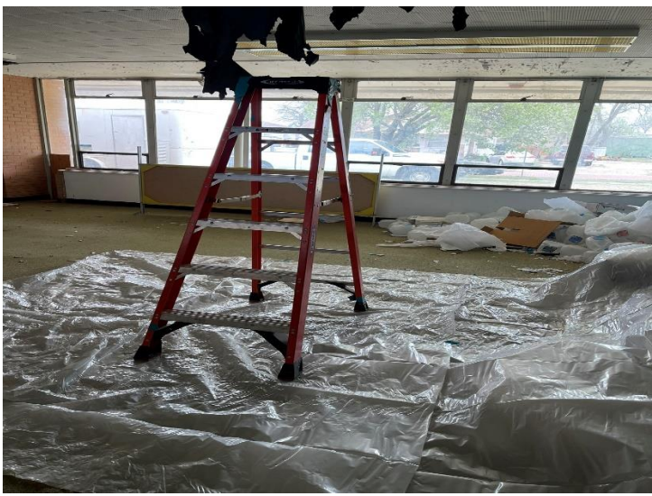
Photo 6: Parkside - South Building - Transit Pannel Abatement
