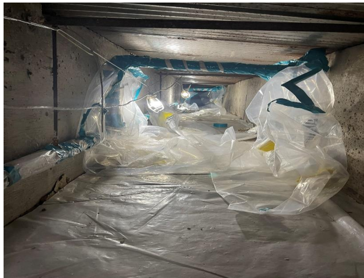
Photo 6: Parkside - in Tunnel - TSI Prep
