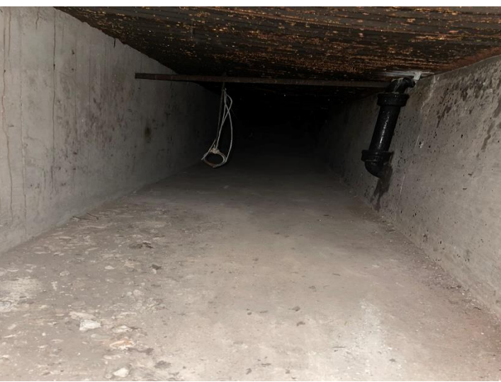
Photo 6: Parkside - in Tunnel - TSI Abated
