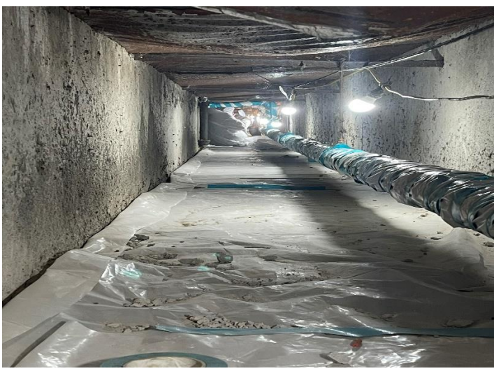
Photo 2: Parkside - in Tunnel - TSI Prep
