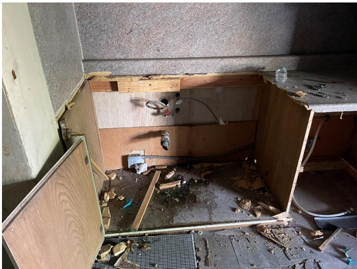
Photo 6: Parkside - East Building - Sink Undercoat Abated
