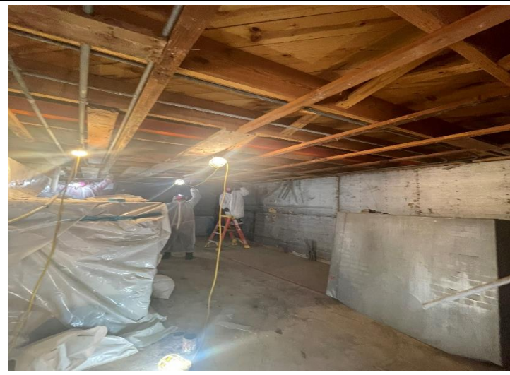
Photo 2: Parkside - North Building - Transit Abatement
