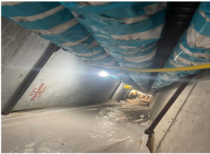
Photo 1: Parkside - in Tunnel - TSI Prep
