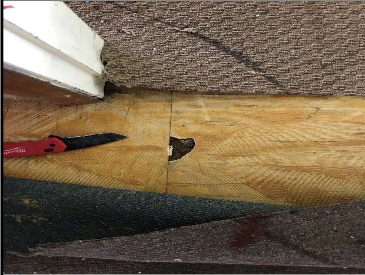
Photo 5: Asbestos Containing Floor Tile Mastic Under Carpet & 12x12 Floor Tile Building 2 Room 7
