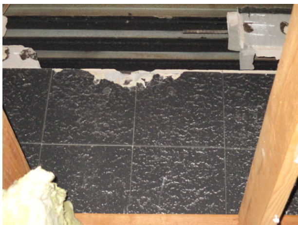
(Homogeneous Area 05) No Asbestos Detected
