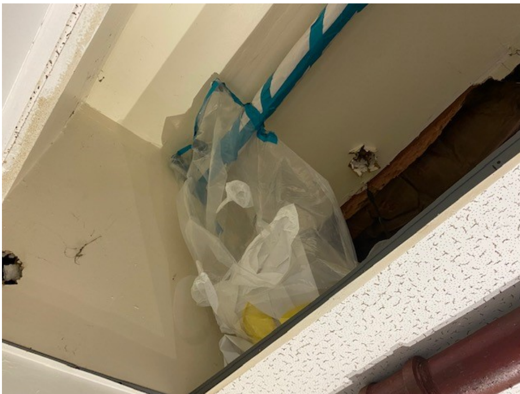
Photo No. 5 – Thermal Pipe & Pipe Fitting Insulation Prepped for Glove-Bag Removal
