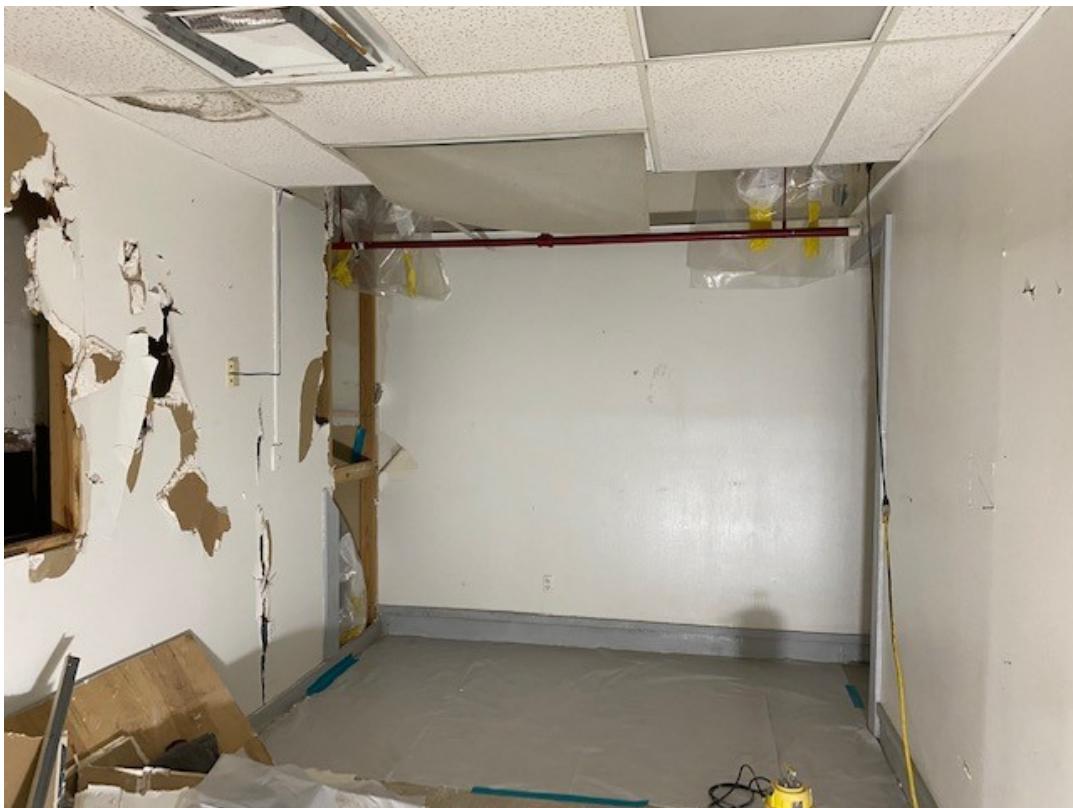
Photo No. 4 – Drop Cloth Installed Below Transite Paneling in Room 116
