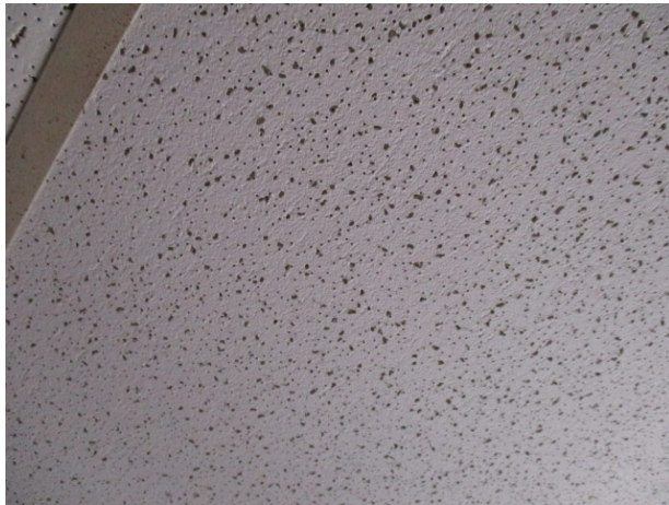
(Homogeneous Area 07) No Asbestos Detected
