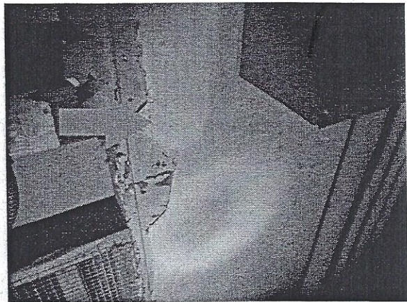
* (Homogeneous Area 08) Asbestos Detected
