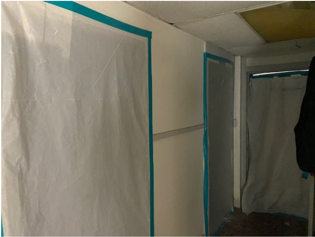
Photo No.1 – Installation of Critical Barriers
