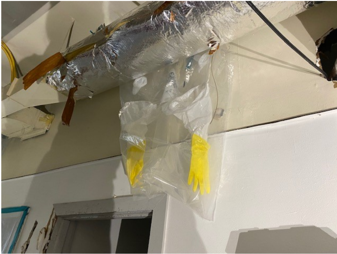
Photo No. 3 – Glove-Bag Prepped and In-Place
