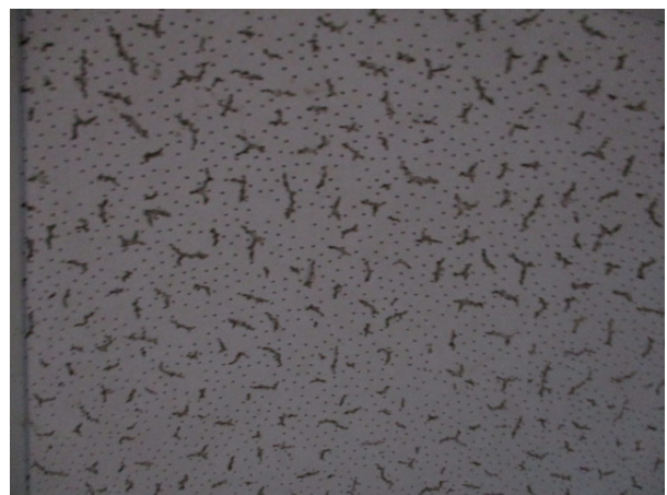
(Homogeneous Area 06) No Asbestos Detected
