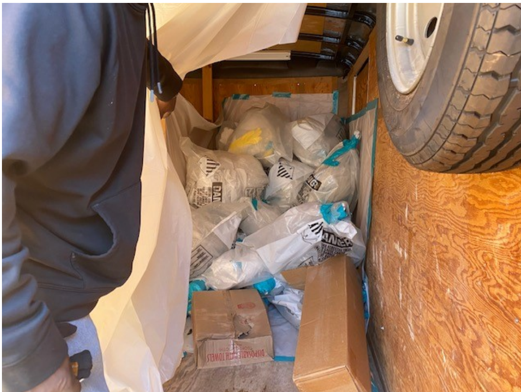
Photo No. 8 – Asbestos Waste Bagged for Transport to Landfill
