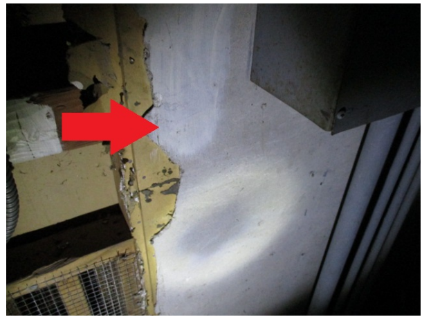
(Homogeneous Area 08) Asbestos Detected
