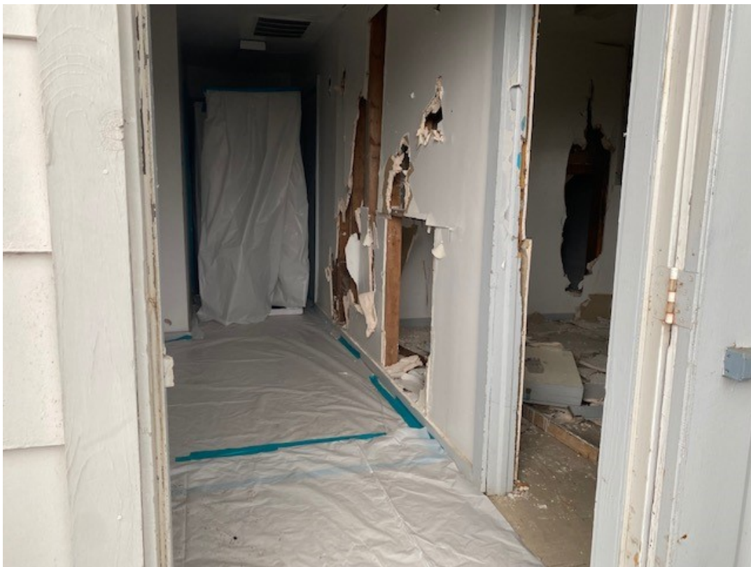
Photo No. 2 – Installation of Drop Cloth, Per Project Design
