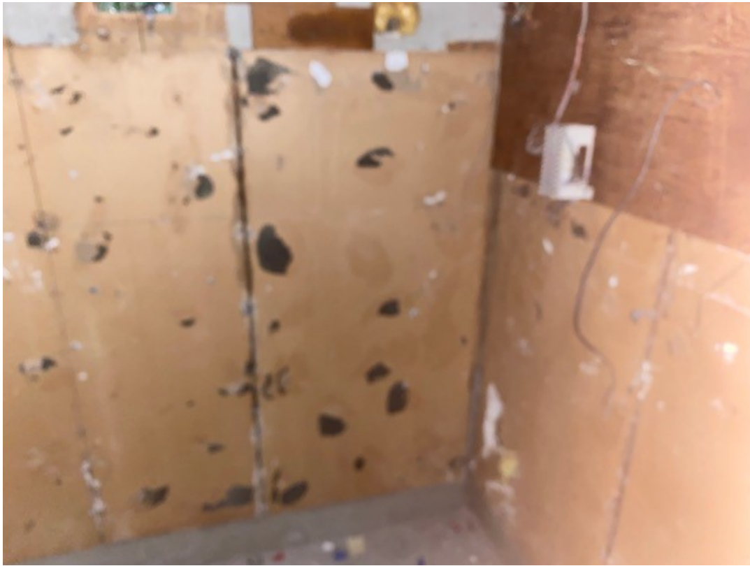
Photo No. 7 – Post Abatement, Removal of Transite Wall Paneling from Room 116
