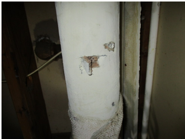
(Homogeneous Area 03) Asbestos Detected
