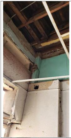
Figure A-12: View of visible masonry demising wall between occupied south area and the remaining unoccupied building.
