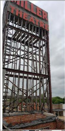
Figure A-16: Steel sign structure that could be removed and mounted at ground level to preserve historic nature of the Theatre.
