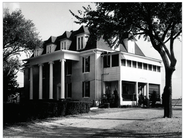
Exterior view of Duke Sanitarium after additions were made to the building in 1911 (236, Helen Holmes Collection, Western History Collections, University of Oklahoma Libraries).
