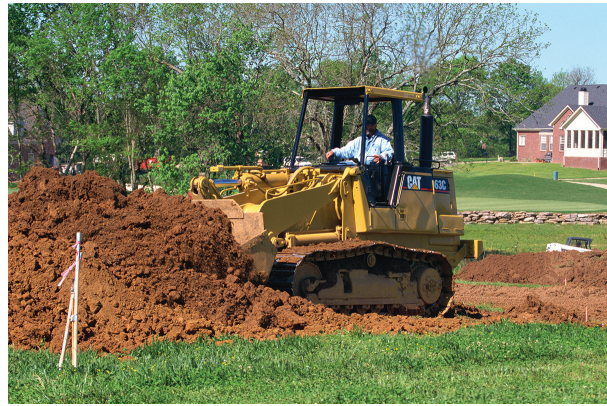
Dirt preparation for building a home Thinkstock Photo
