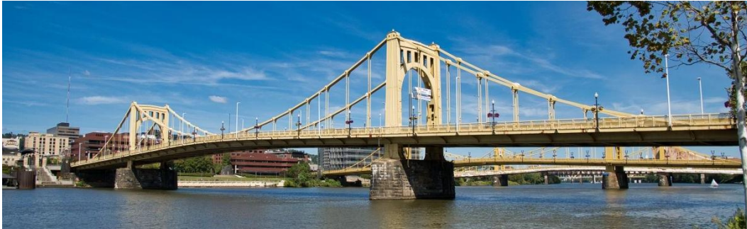
FIGURE 13 – SUSPENSION BRIDGE (ROBERTO CLEMENTE BRIDGE)
