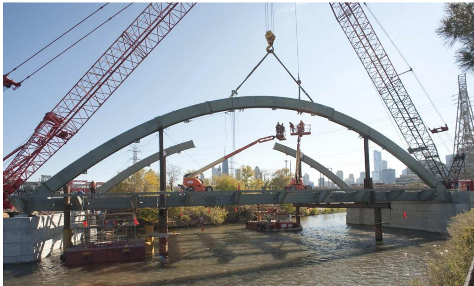
FIGURE 17 – ARCH ERECTION ON FALSEWORK (HALSTED BRIDGE)
