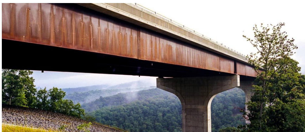
FIGURE 7 – STEEL PLATE GIRDER BRIDGE
