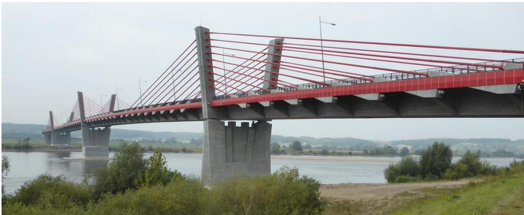
FIGURE 9 – EXTRADOSED BRIDGE (KWIDZYN BRIDGE)
