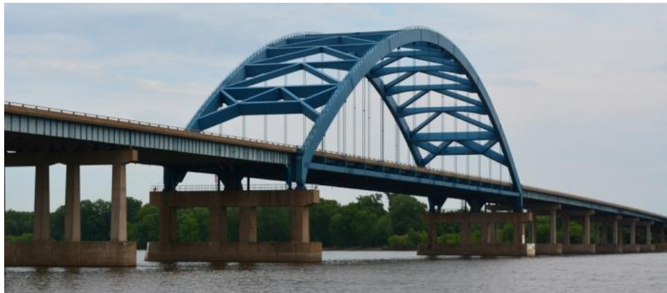
FIGURE 15 – BRIDGE WITH VERTICAL ARCH RIBS (I-280)
