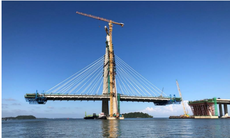
FIGURE 27 – CABLE-STAYED BRIDGE CONSTRUCTION (TEMBURONG BRIDGE)
