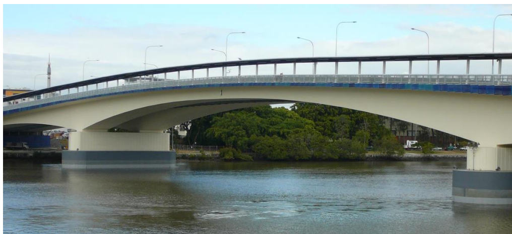
FIGURE 8 – SEGMENTAL CONCRETE BRIDGE (GO BETWEEN BRIDGE)
