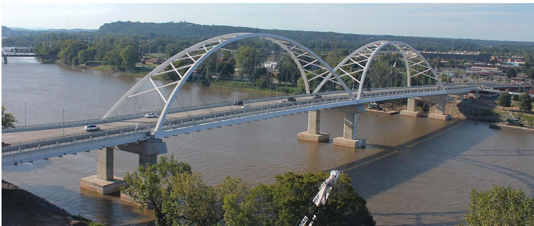
FIGURE 11 – TIED ARCH BRIDGE (BROADWAY BRIDGE)
