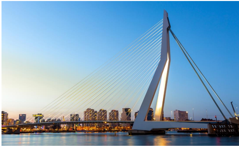
FIGURE 23 – CABLE-STAYED BRIDGE WITH ANGLED TOWER (ERASMUS BRIDGE)
