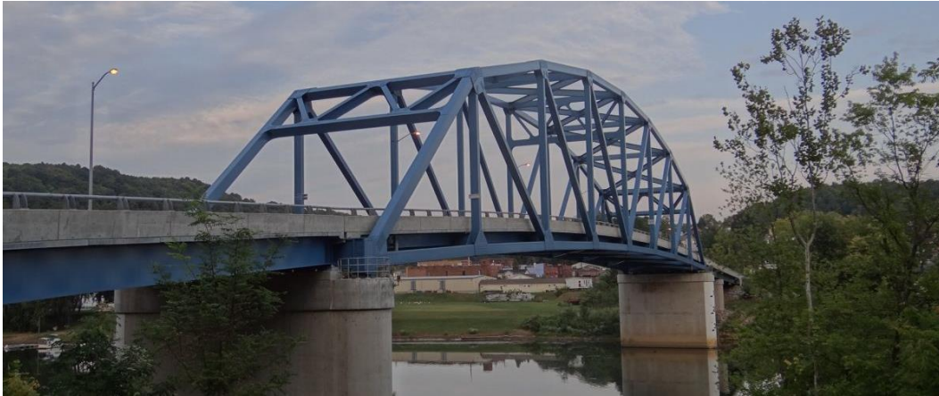
FIGURE 10 – STEEL THROUGH TRUSS BRIDGE (ALBERT GALLATIN MEMORIAL BRIDGE)
