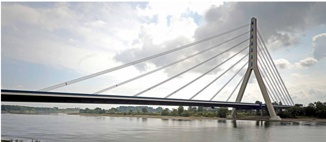
FIGURE 12 – CABLE-STAYED BRIDGE (FLEHE BRIDGE)
