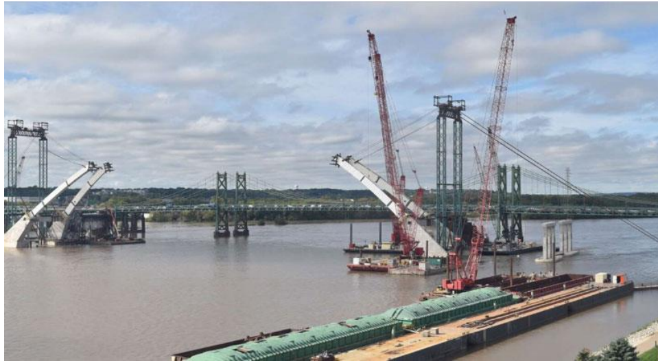
FIGURE 18 – ARCH ERECTION WITH BACK STAYS (I-74)
