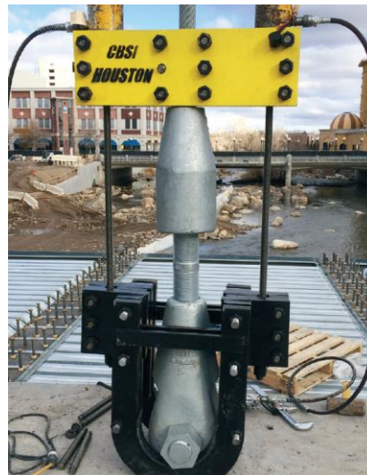
FIGURE 16 – ADJUSTABLE SINGLE STRAND HANGER INSTALLATION
