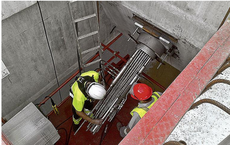
FIGURE 26 – CABLE STAY INSTALLATION
