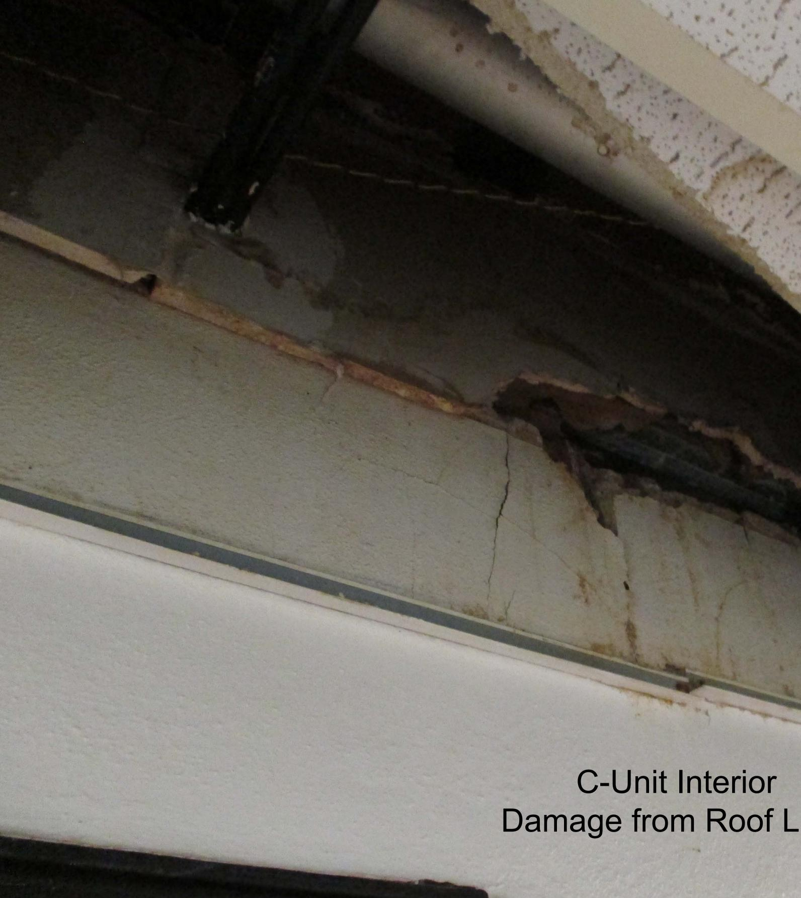
**C-Unit Interior** Damage from Roof Leak
