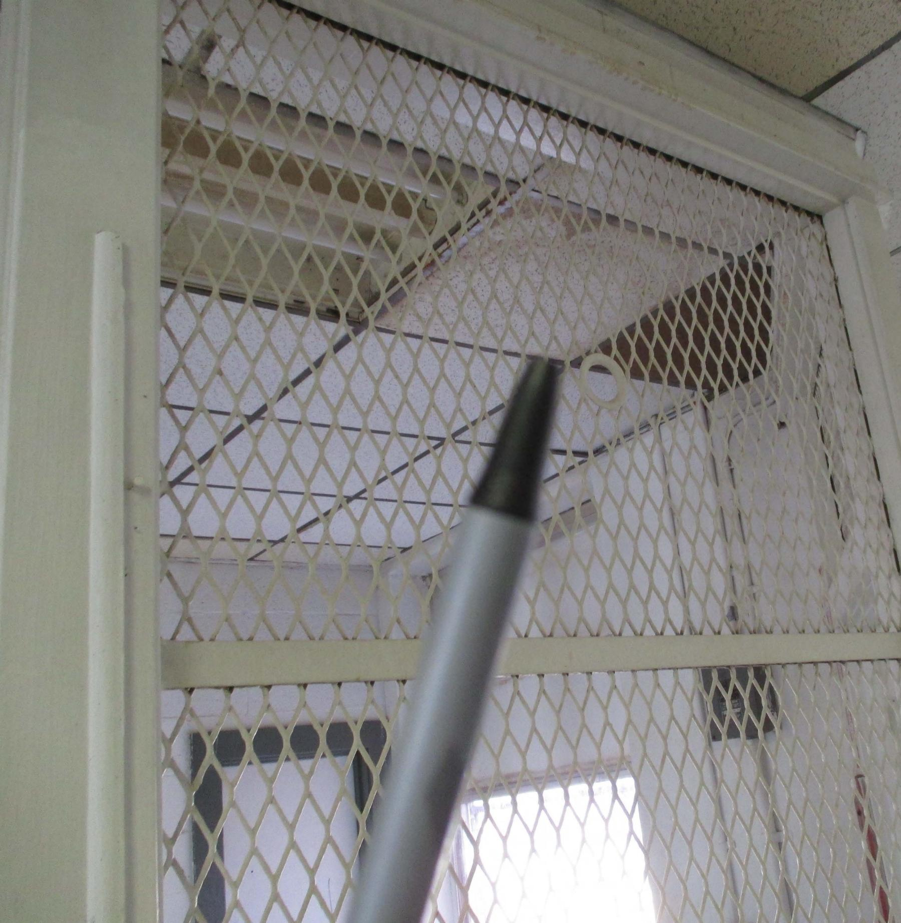
C-Unit Interior Roof Damage with replacing ceiling tiles after each rain
