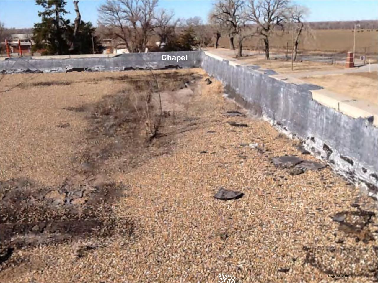
Chapel Roofing missing to decking Chapel Downspout missing from side of building Chapel Roof completely gone. Flashing deteriorated
