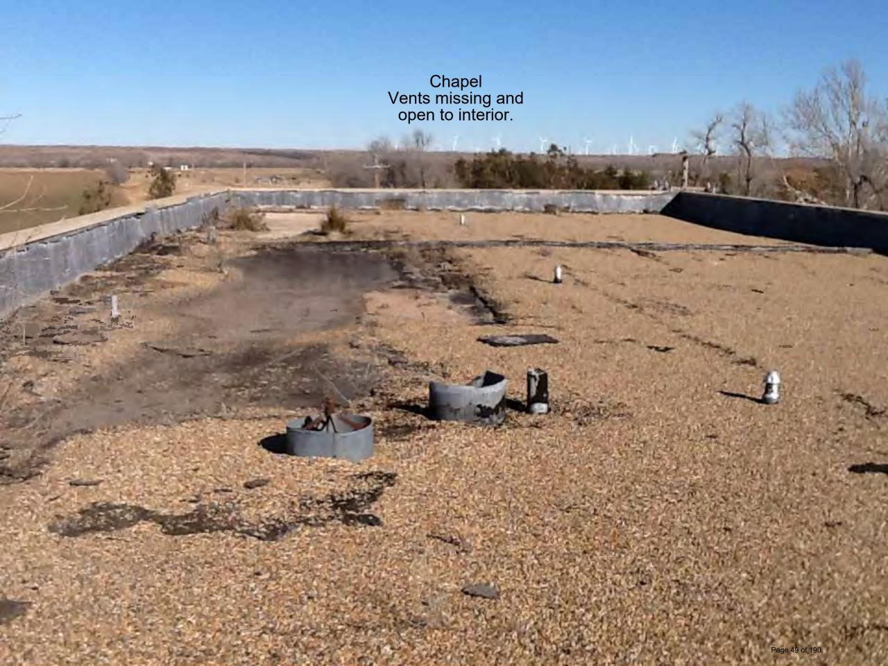
Chapel Looking down the missing vent into the interior Chapel Flashing deteriorated. Roof cap separating
