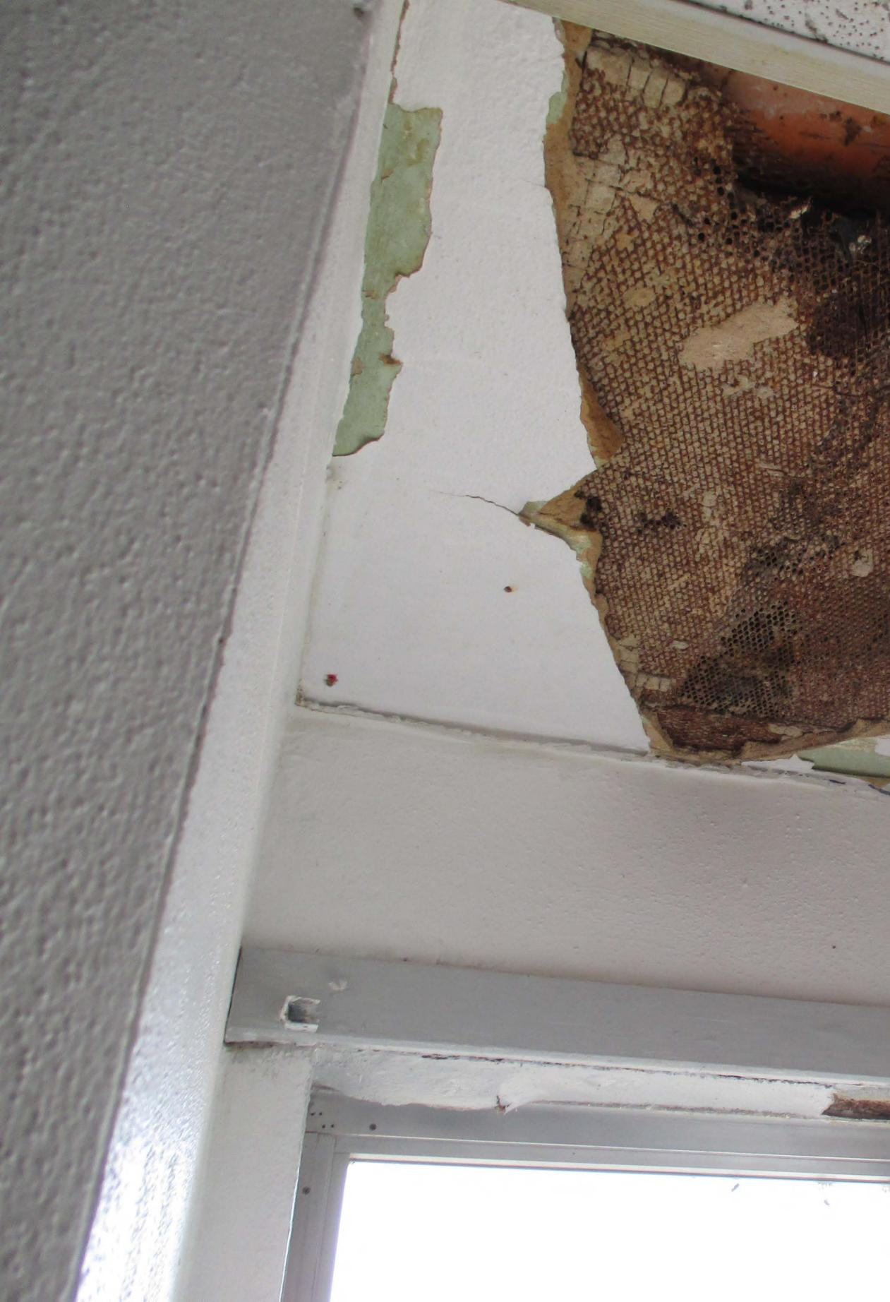
D-Unit Interior Damage from Roof Leak
